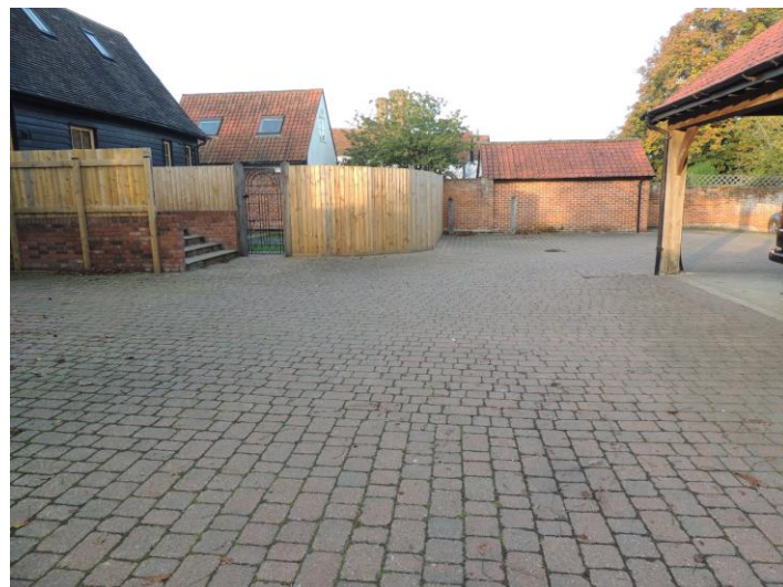
Photo 11: Paved area to west of site
