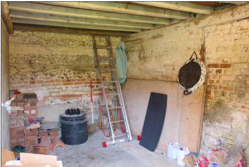
Plate 11: General view of east room of garages, looking northeast. (1m scale)
