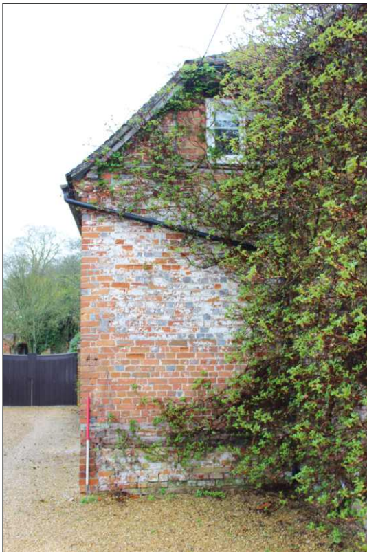
Plate 2: North end of west exterior elevation, looking east. (1m scale)
