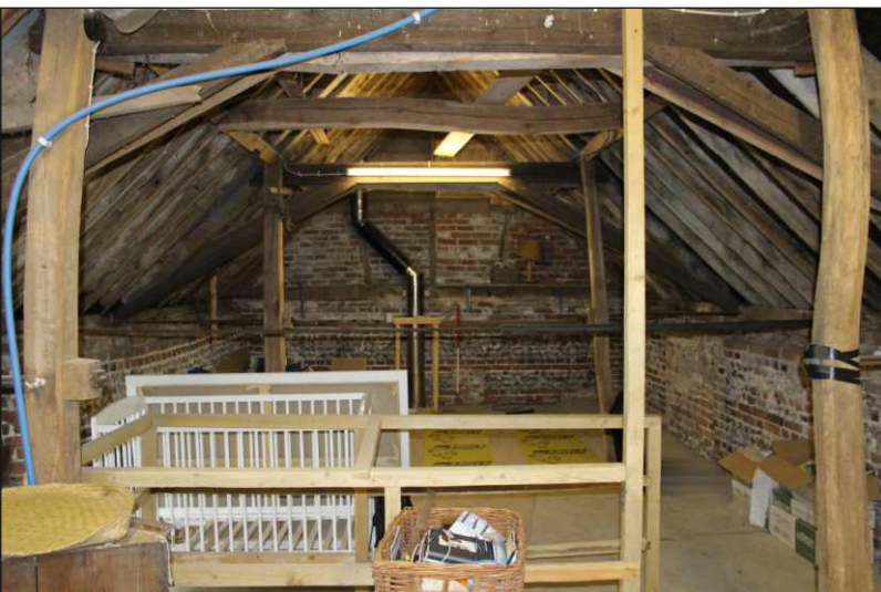
Plate 15: West end of attic, looking west. (1m scale)
