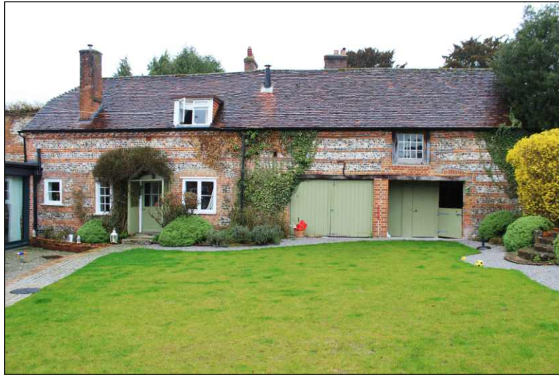
Plate 1: South exterior elevation, looking north. (1m scale)
