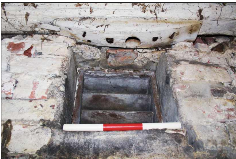
Plate 12: Detail of air vent, with moulded timber, looking east. (0.30m scale)
