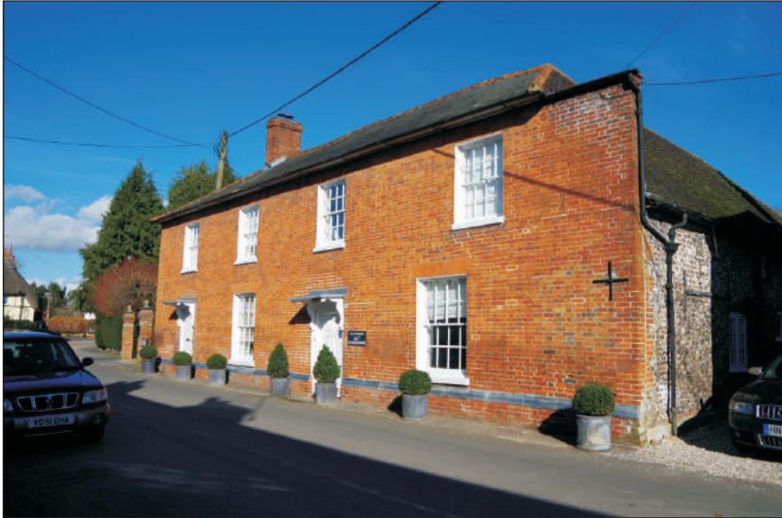
Plate 1: Main, west elevation, looking northeast
