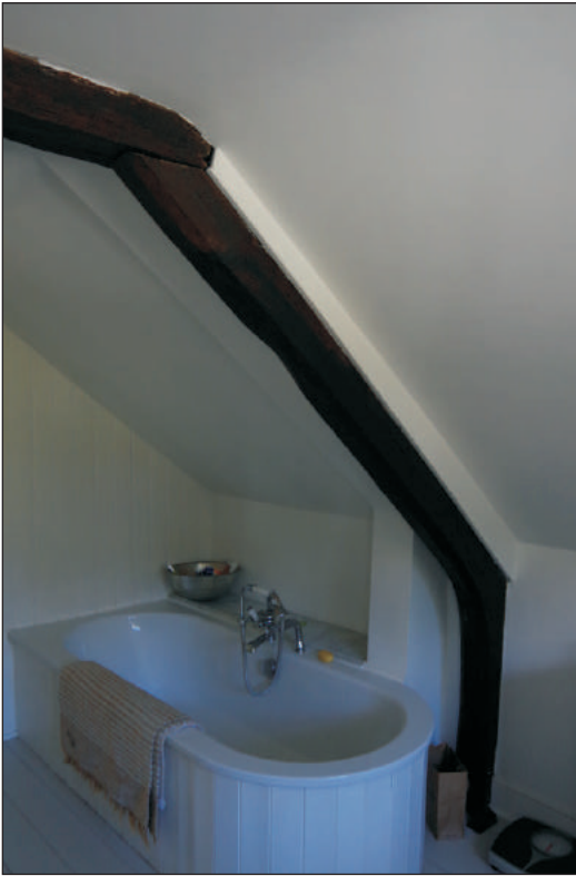
Plate 17: View of jointed cruck in the family bathroom, looking northwest
