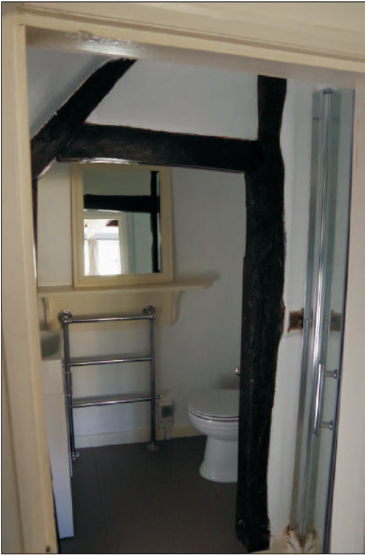
Plate 20: General view of timber framing in en-suite bathroom, looking west-northwest
