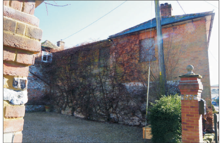
Plate 2: North elevation of the west range, looking southeast
