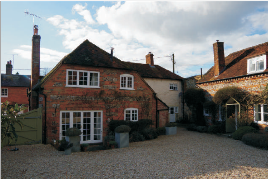
Plate 5: East elevation of the south rangeeast, looking northwest
