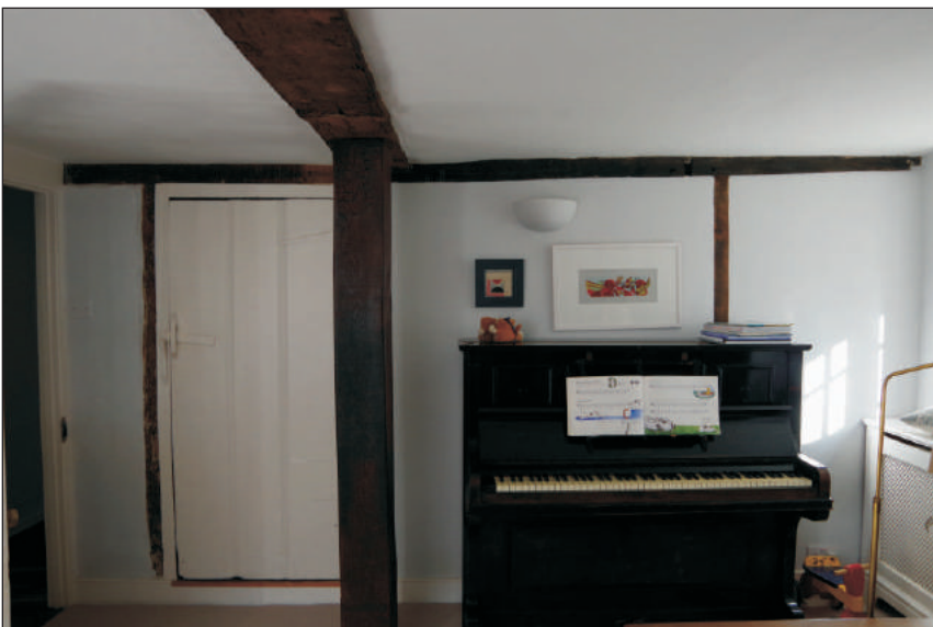
Plate 9: View of timbers in family room, looking east
