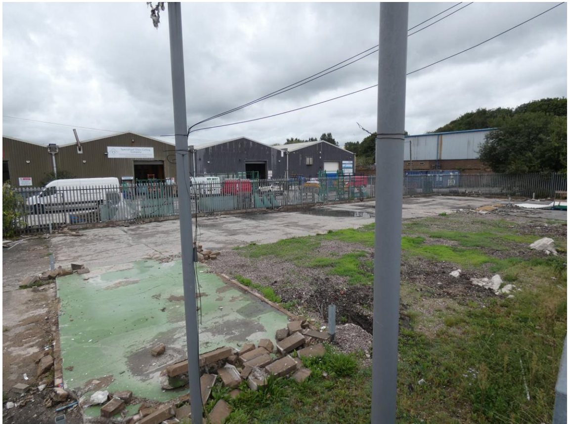
General view of the proposal site, looking towards the east - with Collins Industrial Estate in the background.
