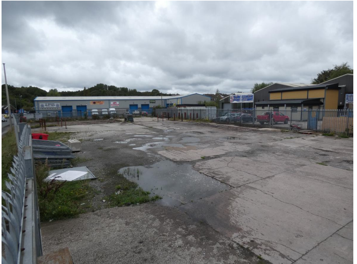
General view of the north end of the proposal site, looking towards the north.
