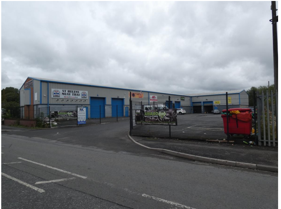
General view of The Barge Business Park directly to the north of the proposal site.
