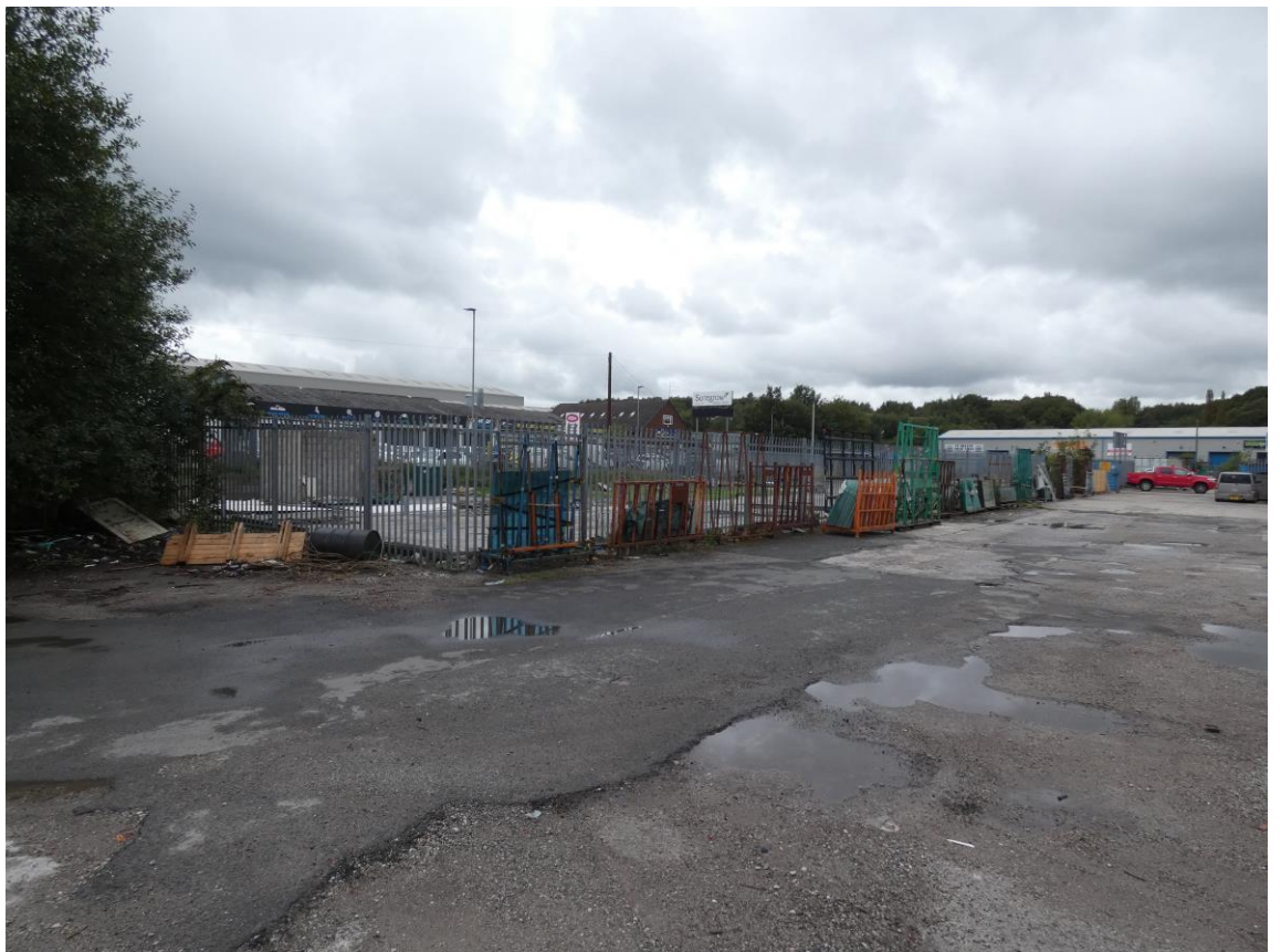
General view of the palisade fencing along the east perimeter of the proposal site with Collins Industrial Estate.
