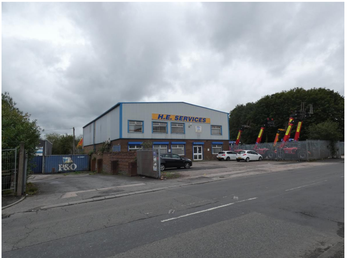
View of the stand-alone unit directly to the south of the proposal site.
