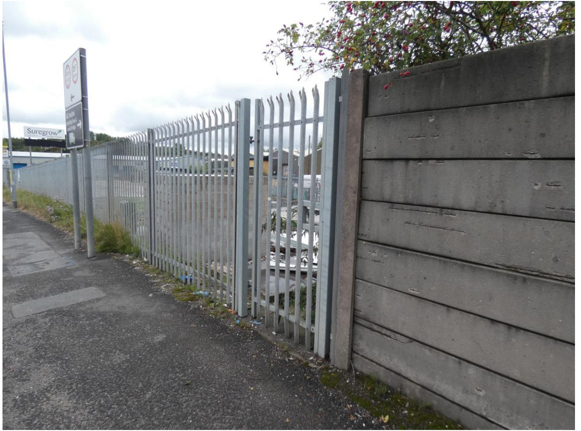
View of the personnel access gate through the front palisade fencing around the south corner of the site.
