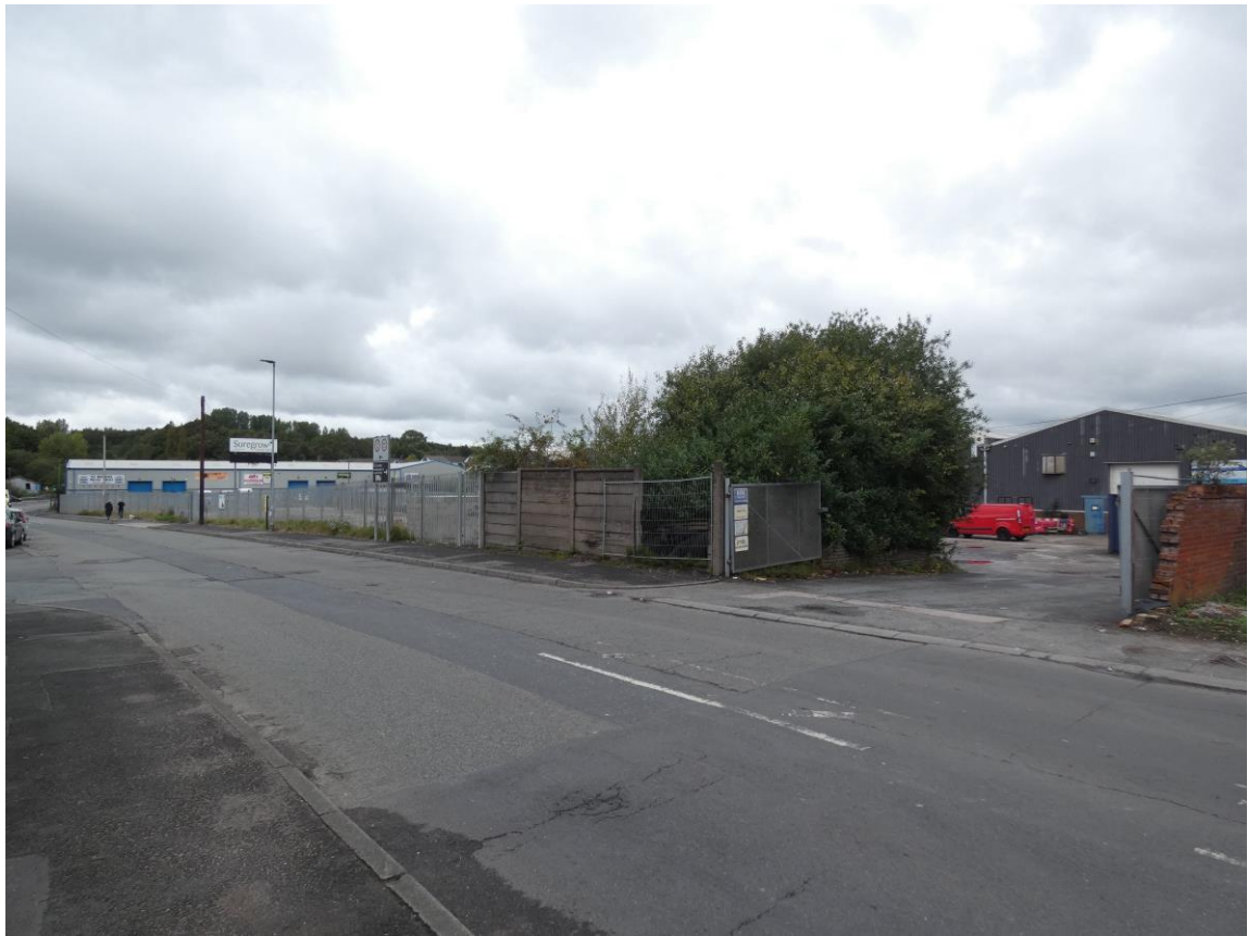
General view of the front of the proposal site, as seen from the west side of Merton Bank Road, looking north.
