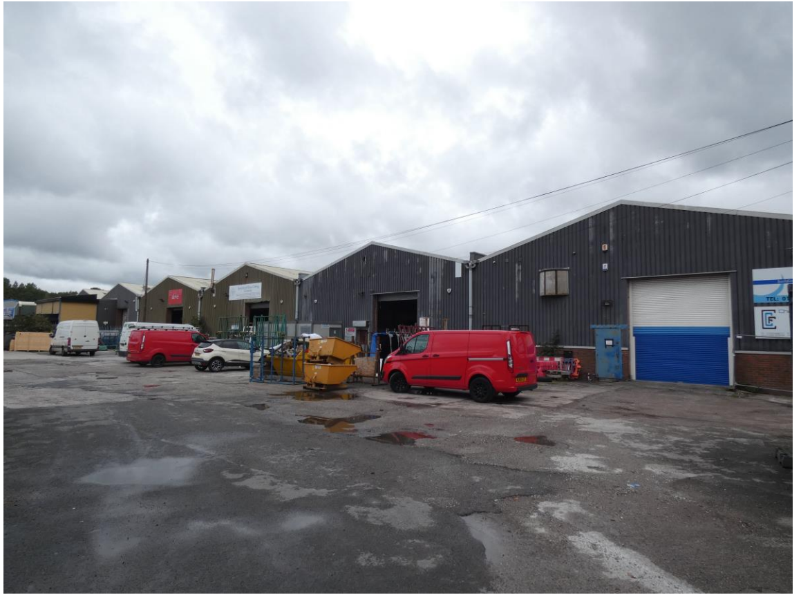
General view of the front elevation of the units comprising 1-6 Collins Industrial Estate, to the east of the site.
