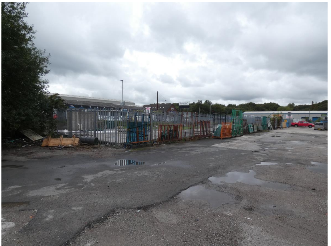
General view of the palisade fencing along the east perimeter of the proposal site with Collins Industrial Estate.
