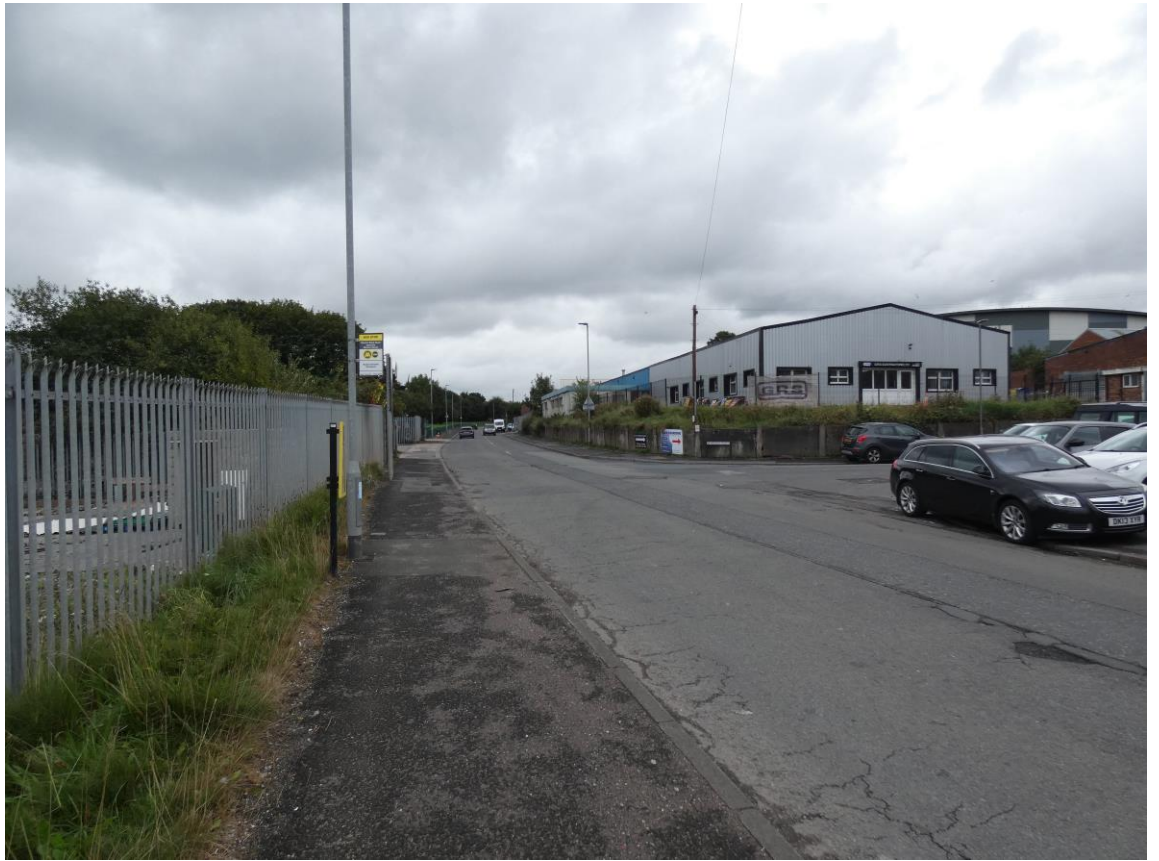
General view of Merton Bank Road, looking south from the proposal site vehicular access gate.
