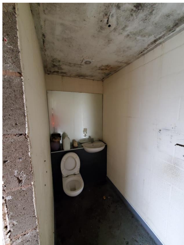
Interior toilet block
