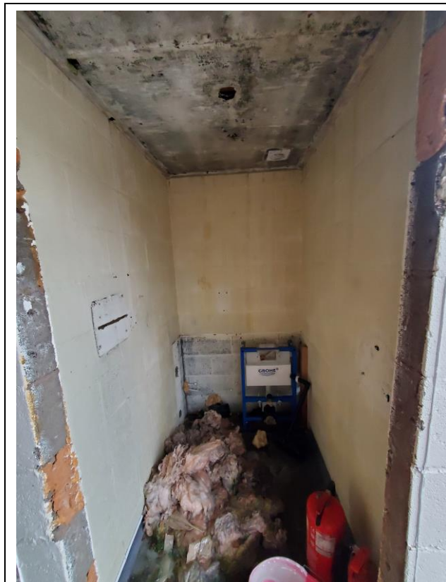
Interior toilet block
