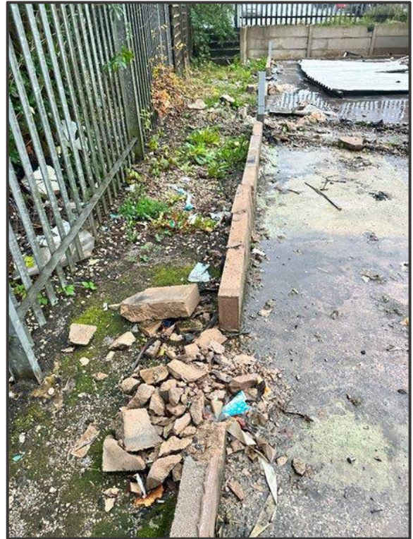
Picture 2. Foundation and heavily compacted hardstanding has likely deflected roots from T1 & T3.
