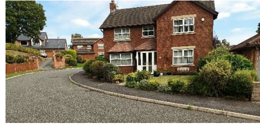
Figure 15 – Existing property on Sandstone Close
