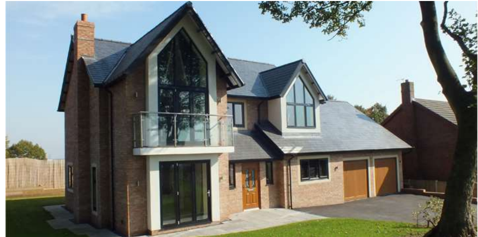
Figure 19 – Existing property at 25 Sandstone Close
