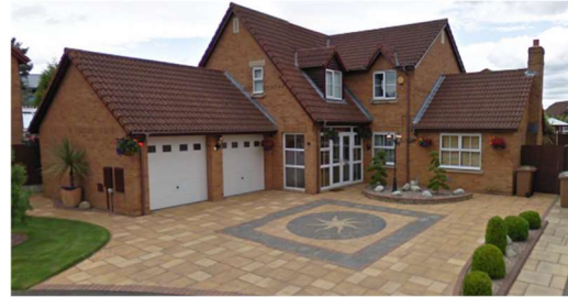
Figure 17 – Existing property on Sandstone Close
