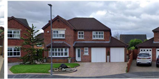
Figure 18 – Existing property on Sandstone Close
