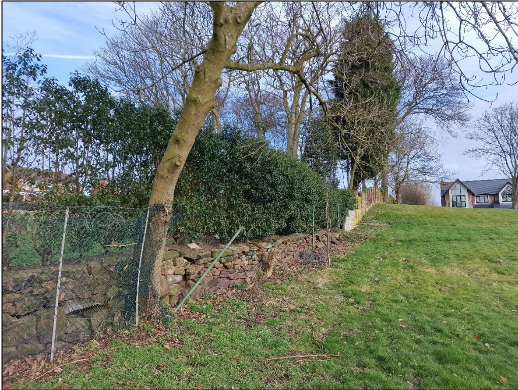
Plate 3 – An image showing the dry-stone wall on the western boundary
