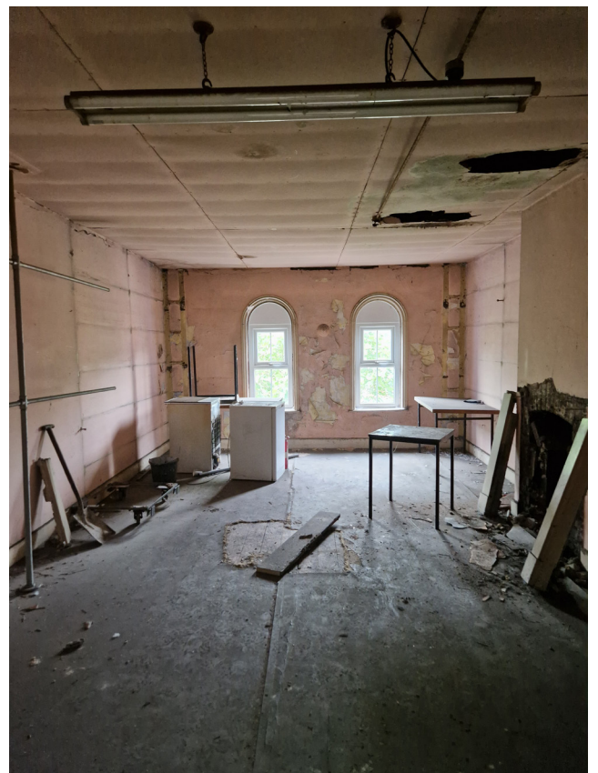
Existing condition of the Saecnd floor bedroom facing the town centre.
