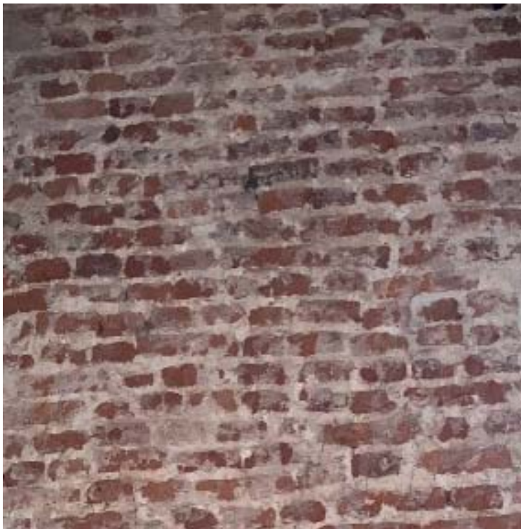
Fig. 2: Exposed wall in the vicinity
