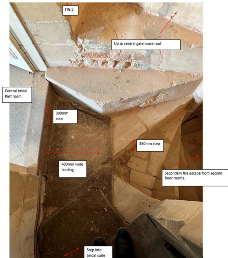
Fig. 1: The configuration of the existing stair
