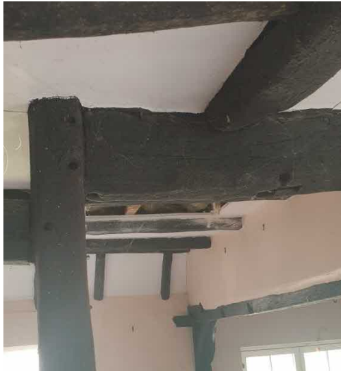
Figure 6, left: Heavy pegged timbers in the kitchen, with heavily scored carpenters marks. Clearly reused from a much older building.
