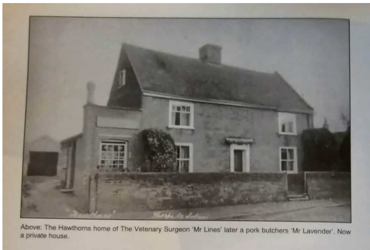
Figure 4: Hawthorns showing the butchers' shop. Note the side access door & parapet before reconstruction
