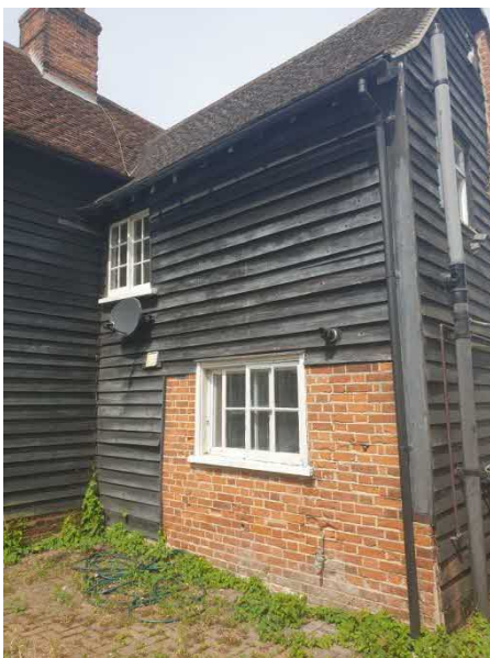
Figure 10, left: The area of weatherboarding to the left of the kitchen window covers the location of a former doorway that appears to have been closed sometime during the 20 th century.
