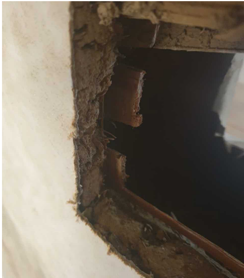
Figure 14: The opened up wall between bedrooms 1 and 2. Sawn softwood laths can be seen here, suggesting a later date than other wall finishes elsewhere in the building. Note the plasterboard finish on the far side of this partition, at the top right of the picture.
