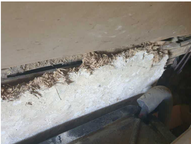
Figure 8, left: In the roof space are panels of riven hardwood laths, coated with daub and finished with a thin lime plaster skim can be seen. This would remain in situ, safely preserved behind new wall finishes.
