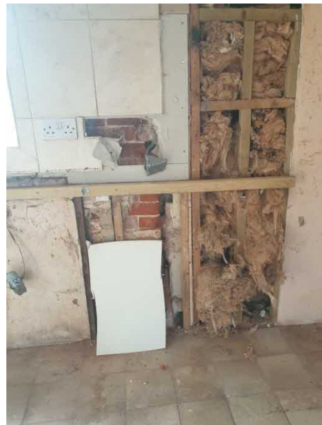
Figure 10, left: The area of weatherboarding to the left of the kitchen window covers the location of a former doorway that appears to have been closed sometime during the 20 th century.
