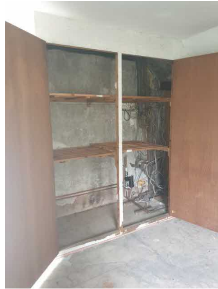
Figure 12, left: Ledged and boarded bathroom door. Figure 13, right: The large airing cupboard in the bathroom.
