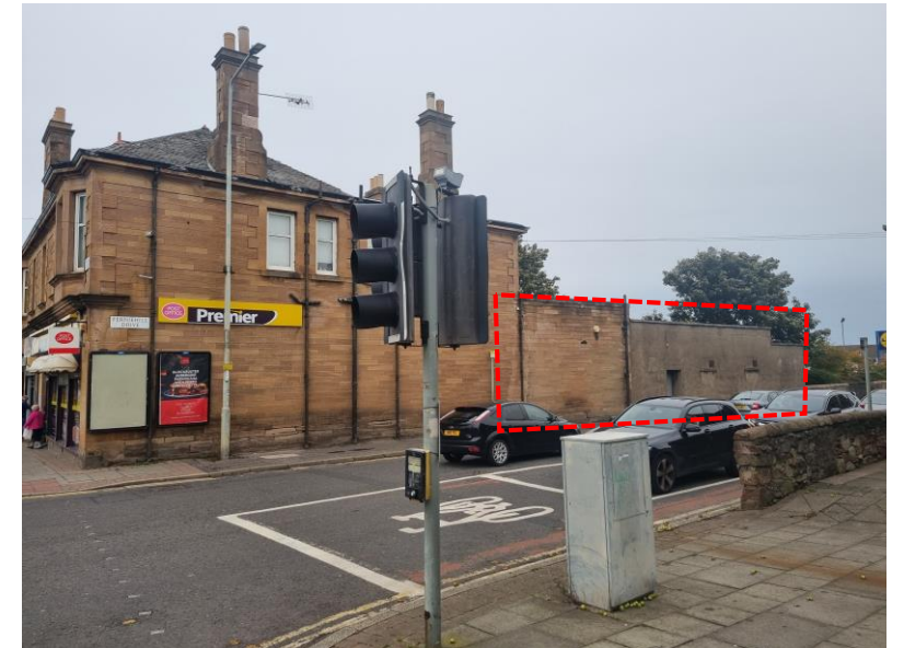
Photo 2. Side elevation along Fernieside Drive
