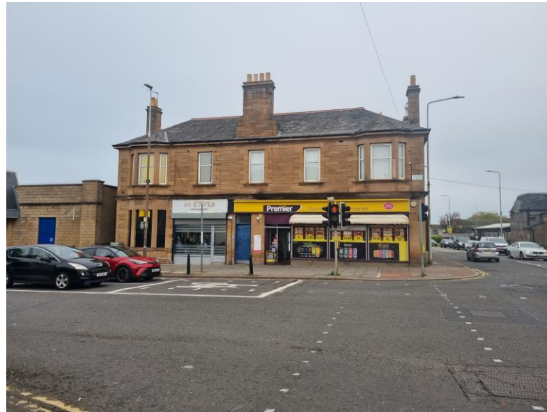
Photo 1. Shop frontage to Drum Street
