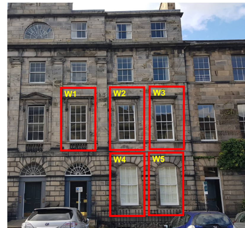
PHOTO OF FRONT ELEVATION INDICATING APPROVED WINDOW REPLACEMENTS
