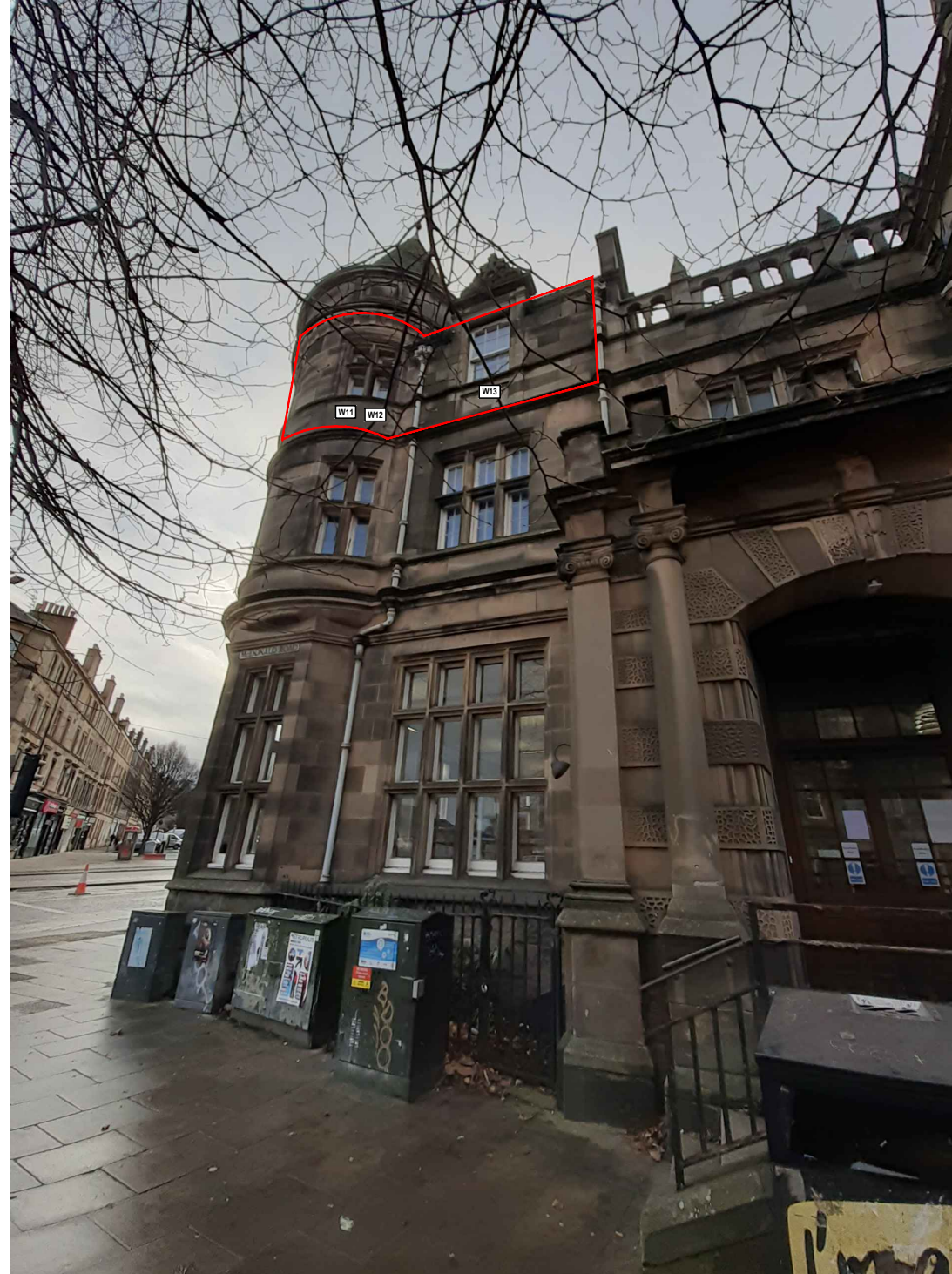
PHOTO OF SIDE ELEVATION (NTS) 41 2F HADDINGTON PLACE, EH7 4AG
