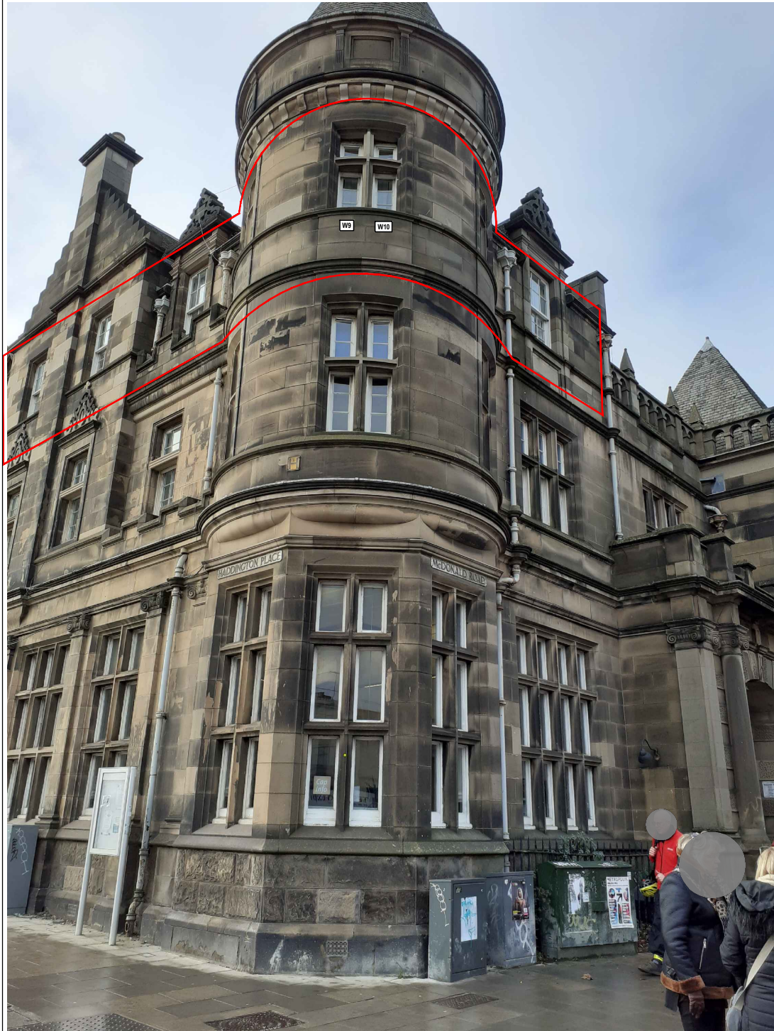
PHOTO OF CORNER ELEVATION (NTS) 41 2F HADDINGTON PLACE, EH7 4AG
