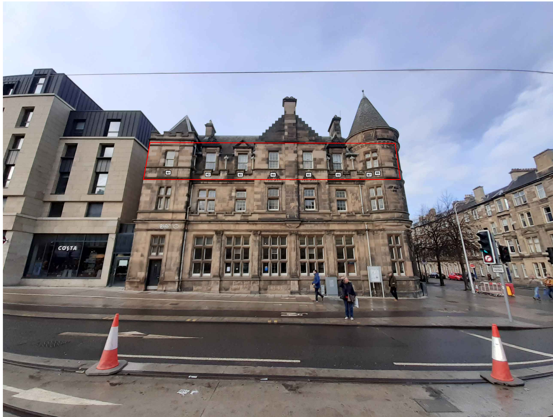
PHOTO OF FRONT ELEVATION (NTS) 41 2F HADDINGTON PLACE, EH7 4AG
