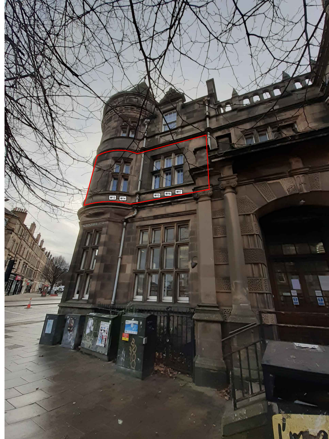
PHOTO OF SIDE ELEVATION (NTS) 41 1F HADDINGTON PLACE, EH7 4AG
