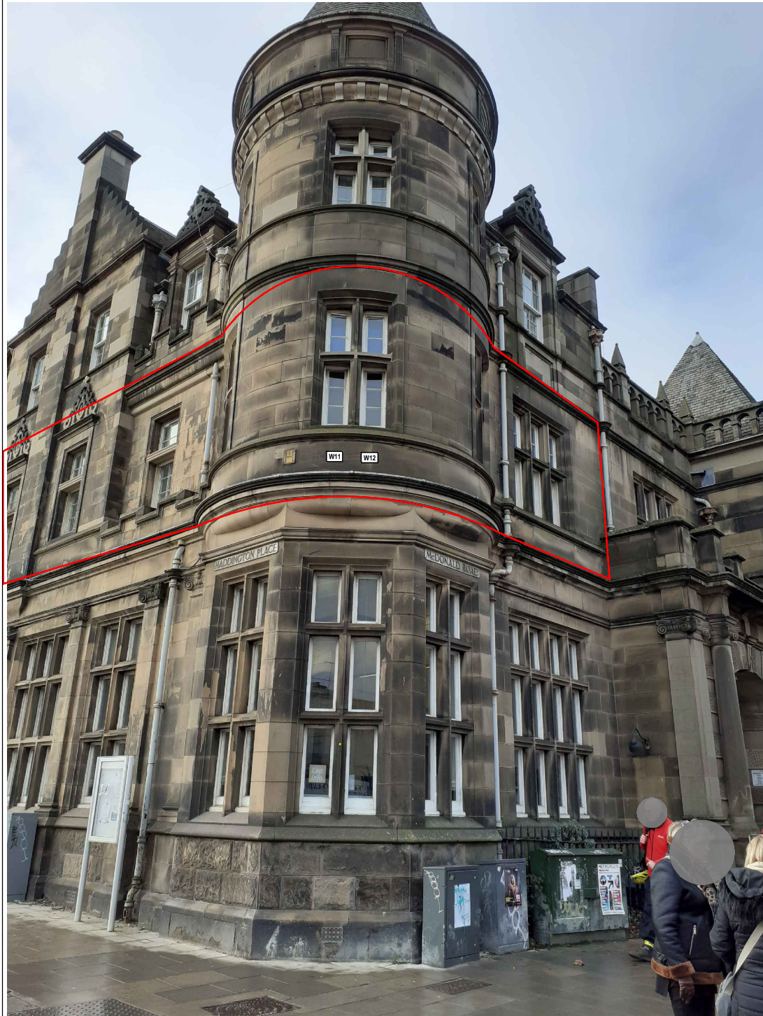
PHOTO OF CORNER ELEVATION (NTS) 41 1F HADDINGTON PLACE, EH7 4AG
