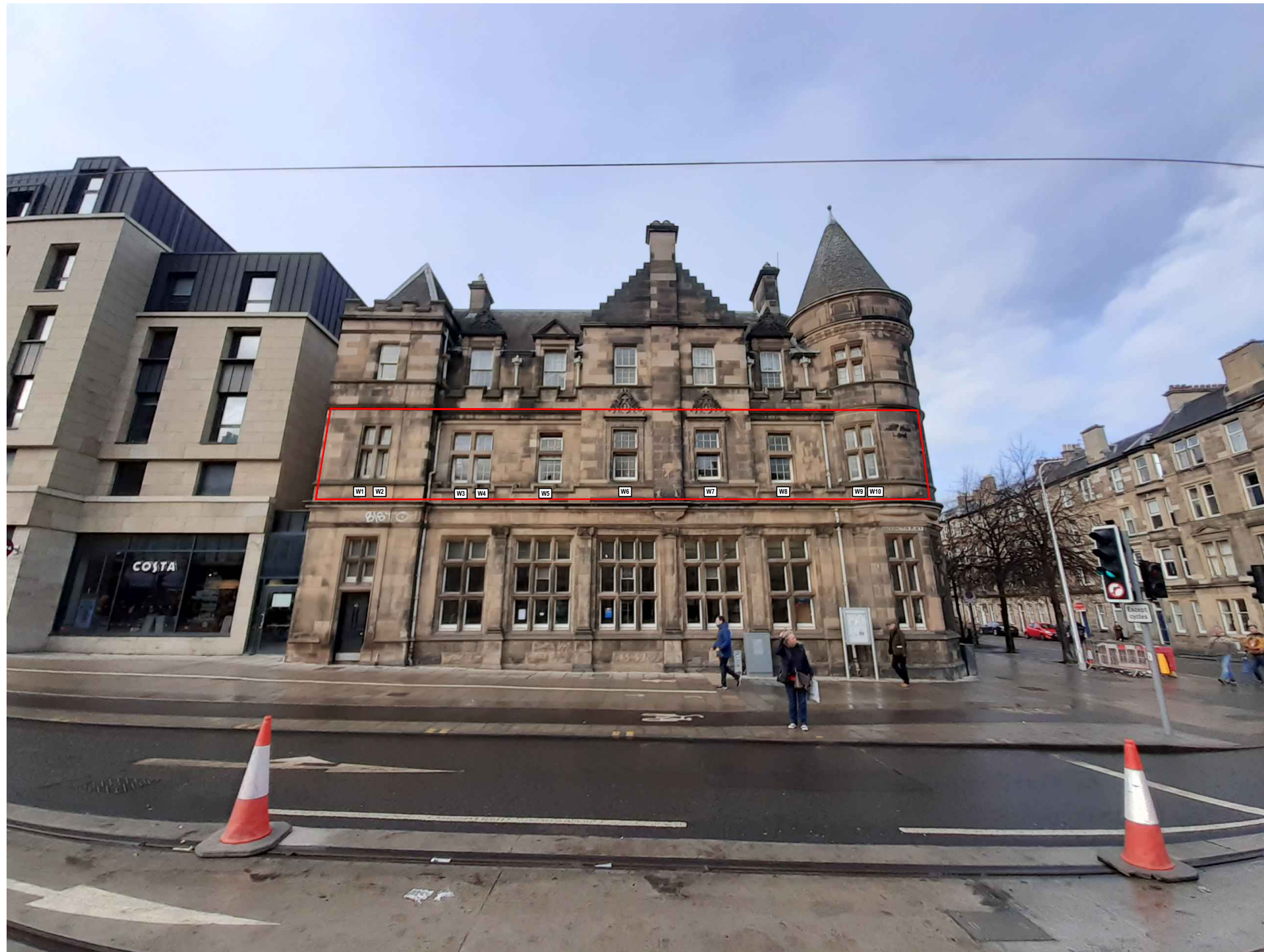
PHOTO OF FRONT ELEVATION (NTS) 41 1F HADDINGTON PLACE, EH7 4AG
