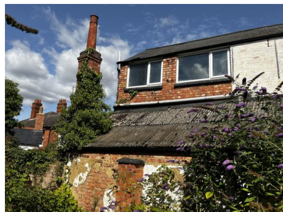
Front façade looking East
