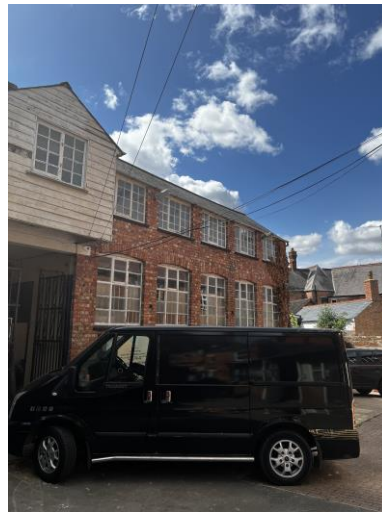
Front façade looking West
