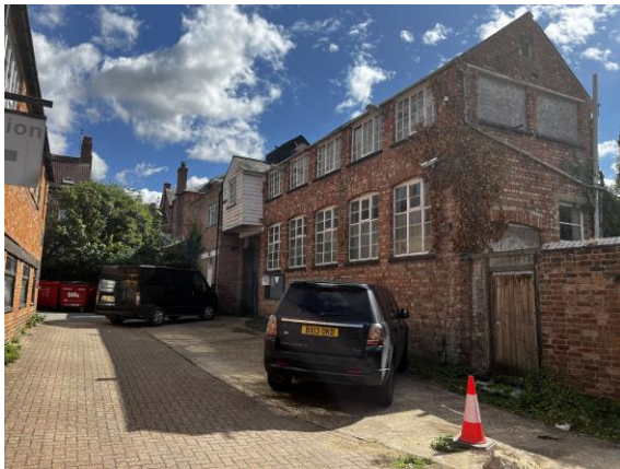
Front façade looking East
