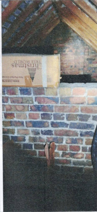
Photo 5 – showing the somewhat cluttered main roof void
