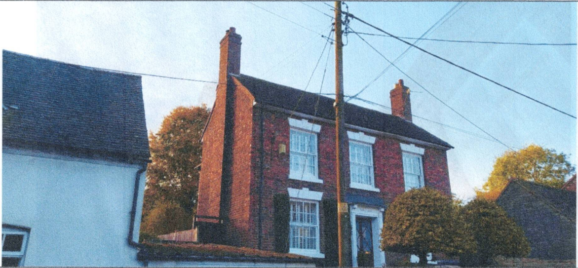
Photo 1 – shows the east and south-facing elevations.
