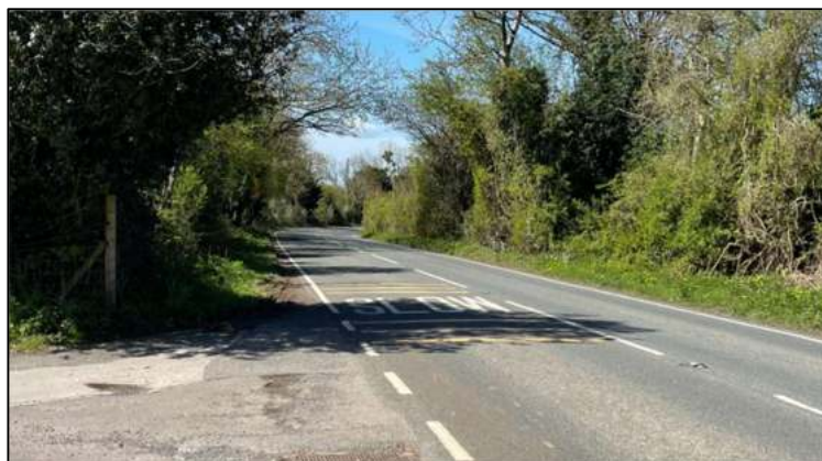
FIGURE 5.: CLEVEDON ROAD LOOKING WEST FROM UNCLASSIFIED ROAD
