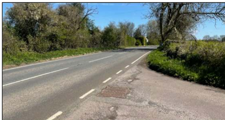
FIGURE 6.: CLEVEDON ROAD LOOKING EAST FROM UNCLASSIFIED ROAD
