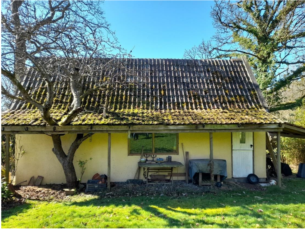
Photograph 2: Eastern aspect of garage with an apple tree growing through the covered porch.
