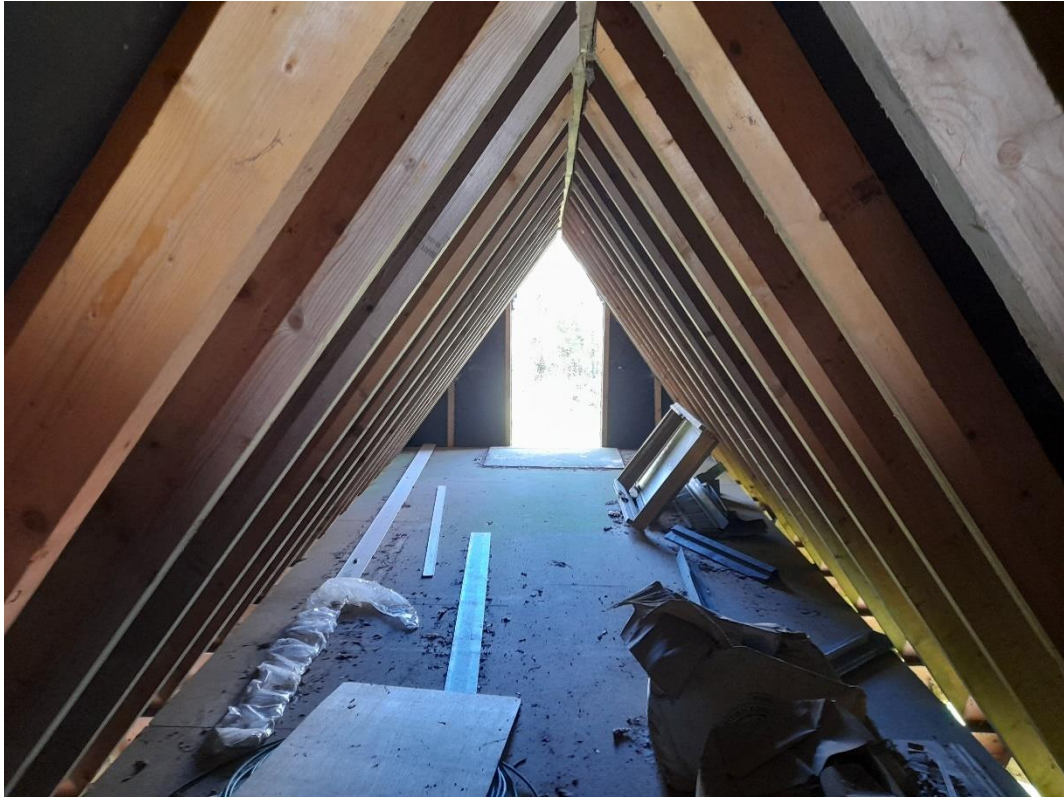
Photograph 6: Roof void open at northern end, with gaps at the eaves along the western and eastern aspects.
