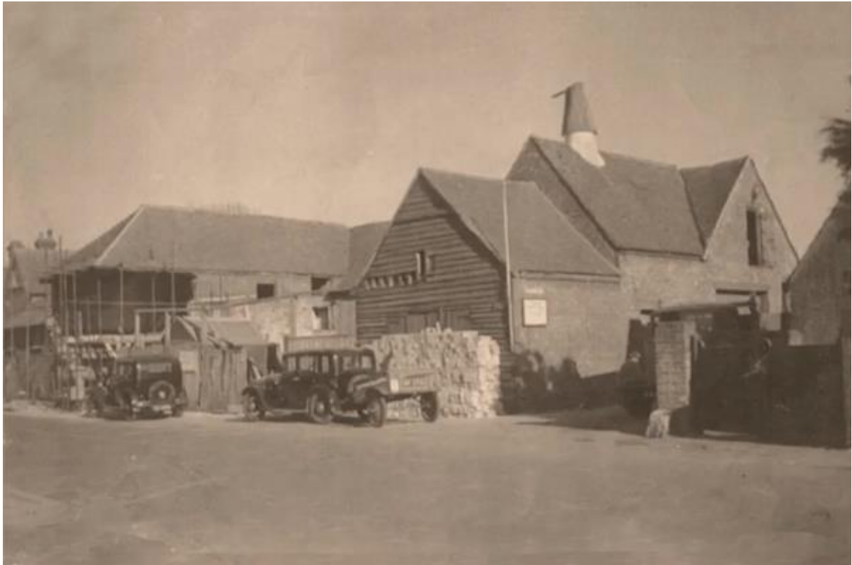
The Malt Hall and adjacent buildings from New Street-date unknown but believed to be 1948
