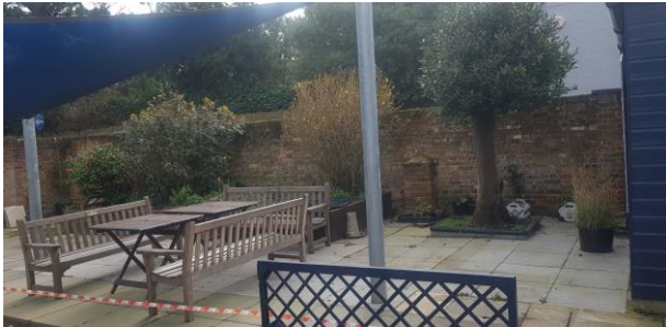
Views within Courtyard
