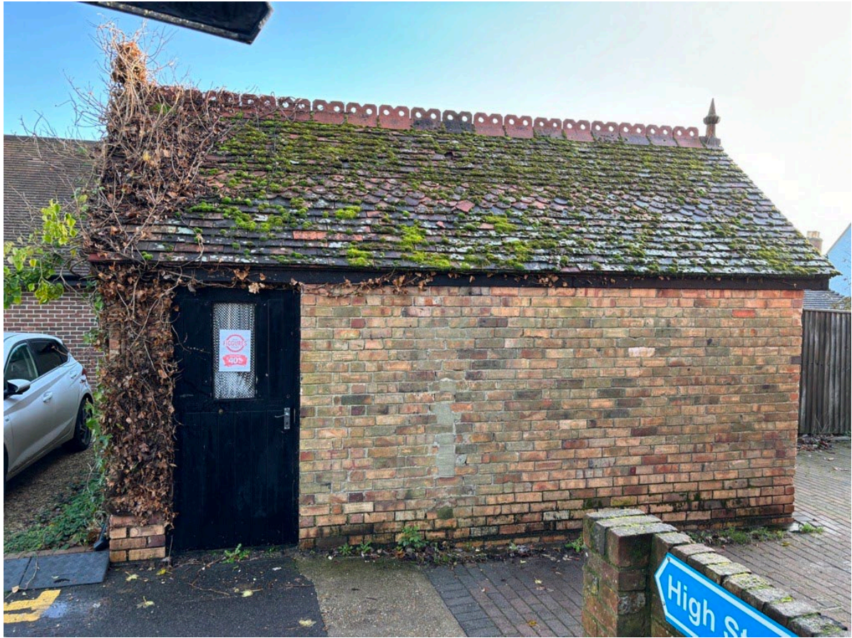
Figure 2. Side view of garage from walkthrough.
