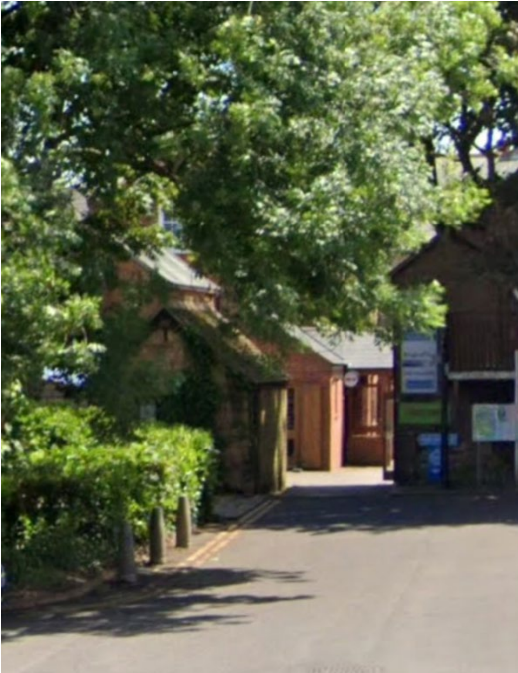
Figure 1 View of Garage from Cannon Street short stay car park.
