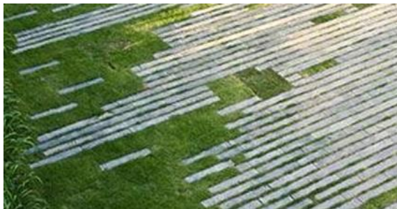
Figure 22 - Contemporary grasscrete to residential entrance and driveway.
