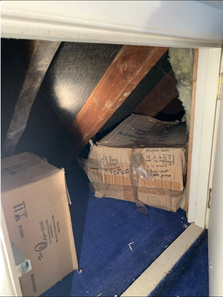
Photograph 5: Lower loft void.
