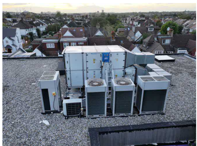
4. Existing plant from east
