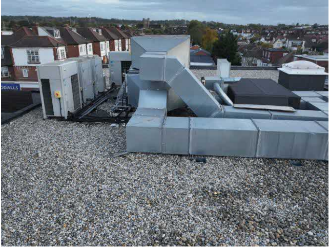
5: Existing roof plant from north
