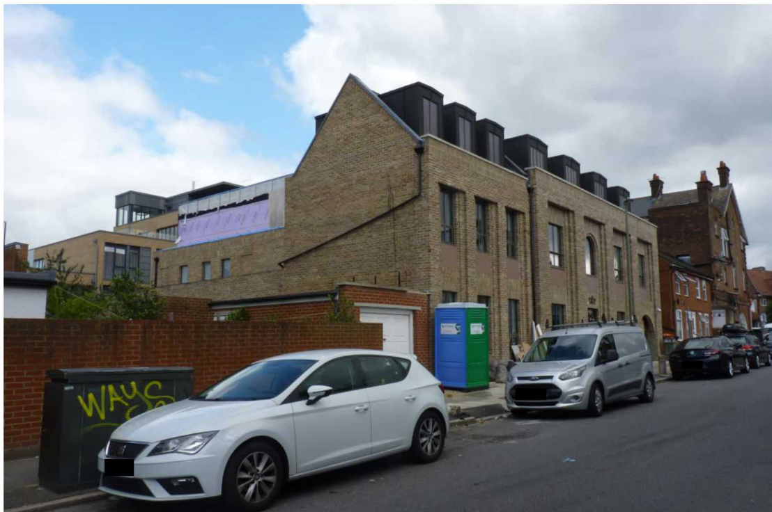
View of front elevation to St George's Road from West with neighbouring 5 storey scheme to North
