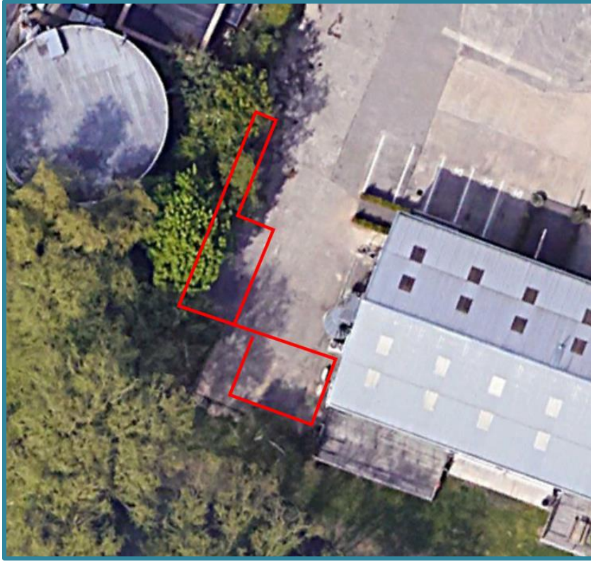
Figure 3 Site outline superimposed on Google Earth image showing site entirely on existing concrete slab.
