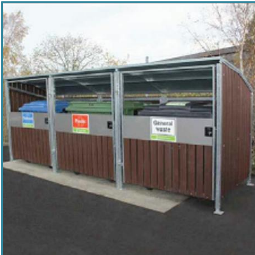
Figure 7 Typical bin store – note it is raised above the slab on legs.
