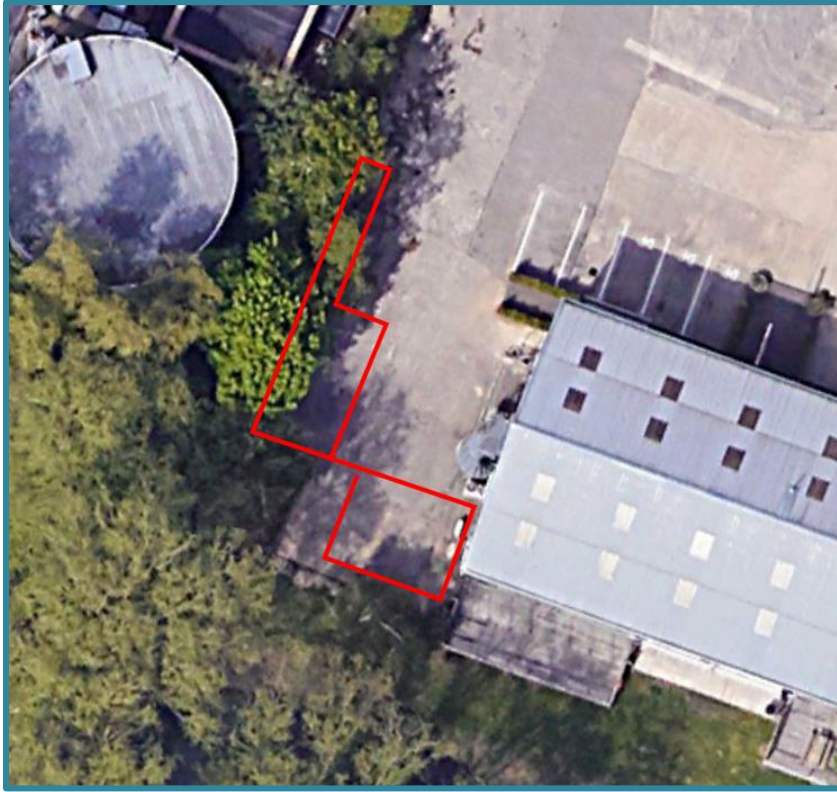
Figure 3 Site outline superimposed on Google Earth image showing site entirely on existing concrete slab.
