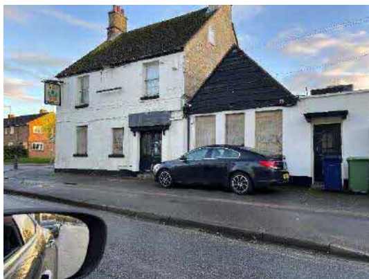
Old Road Elevation
