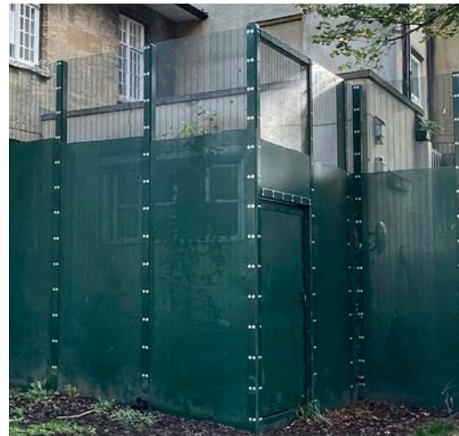
Example of fencing found across the site
