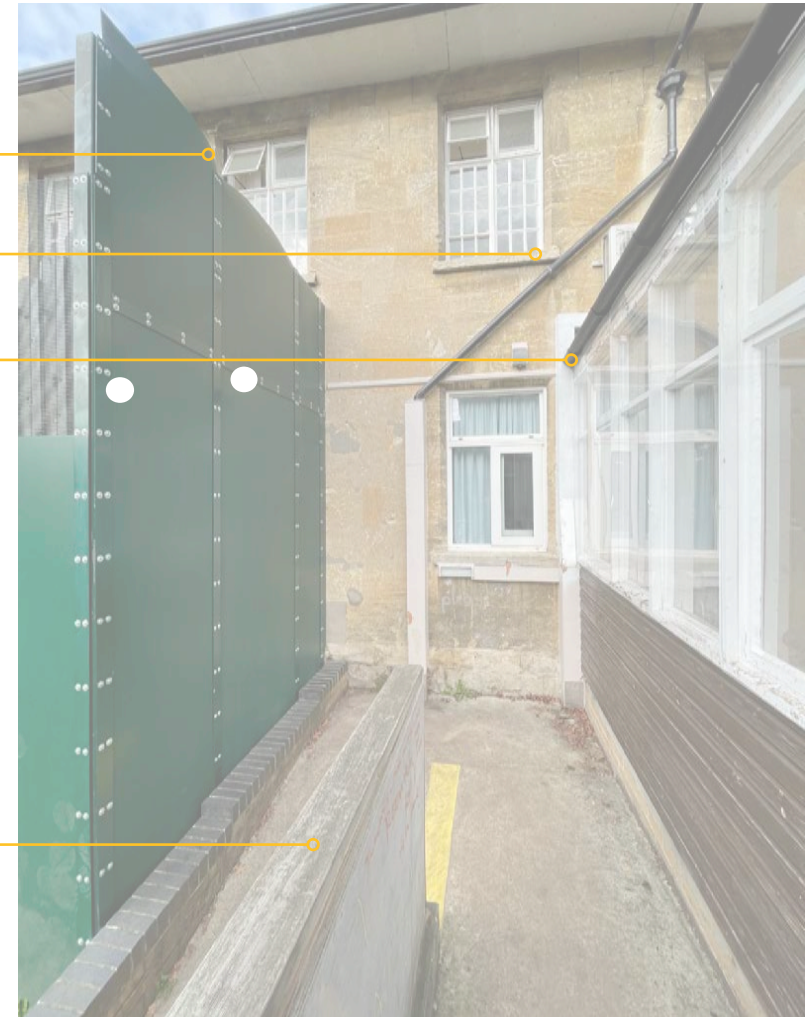
▲ Example of fencing found across the site
