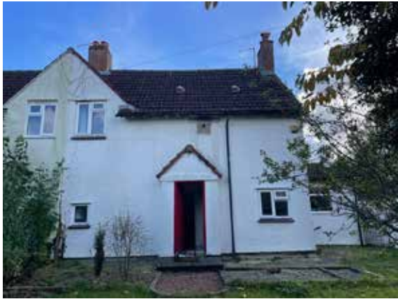
View from Churchill Place
