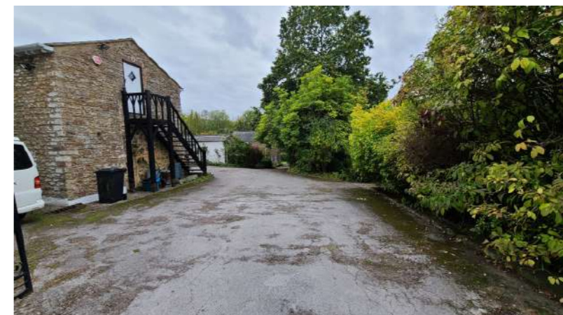
FIG 16. Driveway entrance from Old Monmouth road
