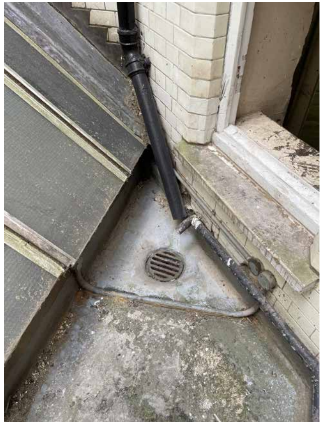
Plate 27 Lightwell drain, south side (DIA)
