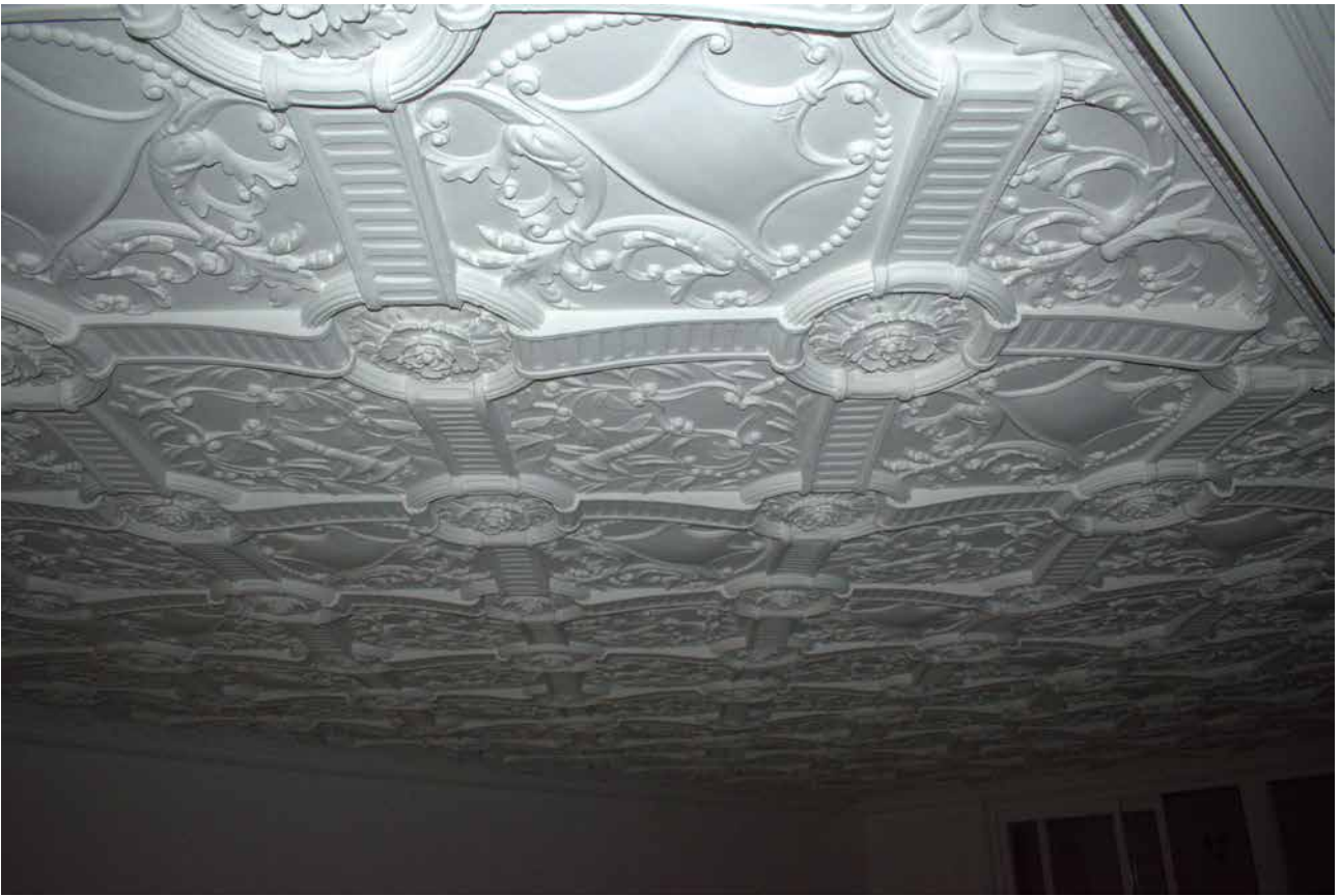
Plate 10 Fibrous plasterwork ceiling to double height space (DIA)
