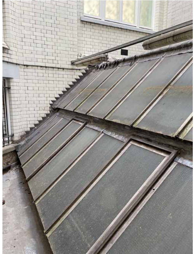
Plate 25 Glazed roof in lightwell (south side) (DIA)
