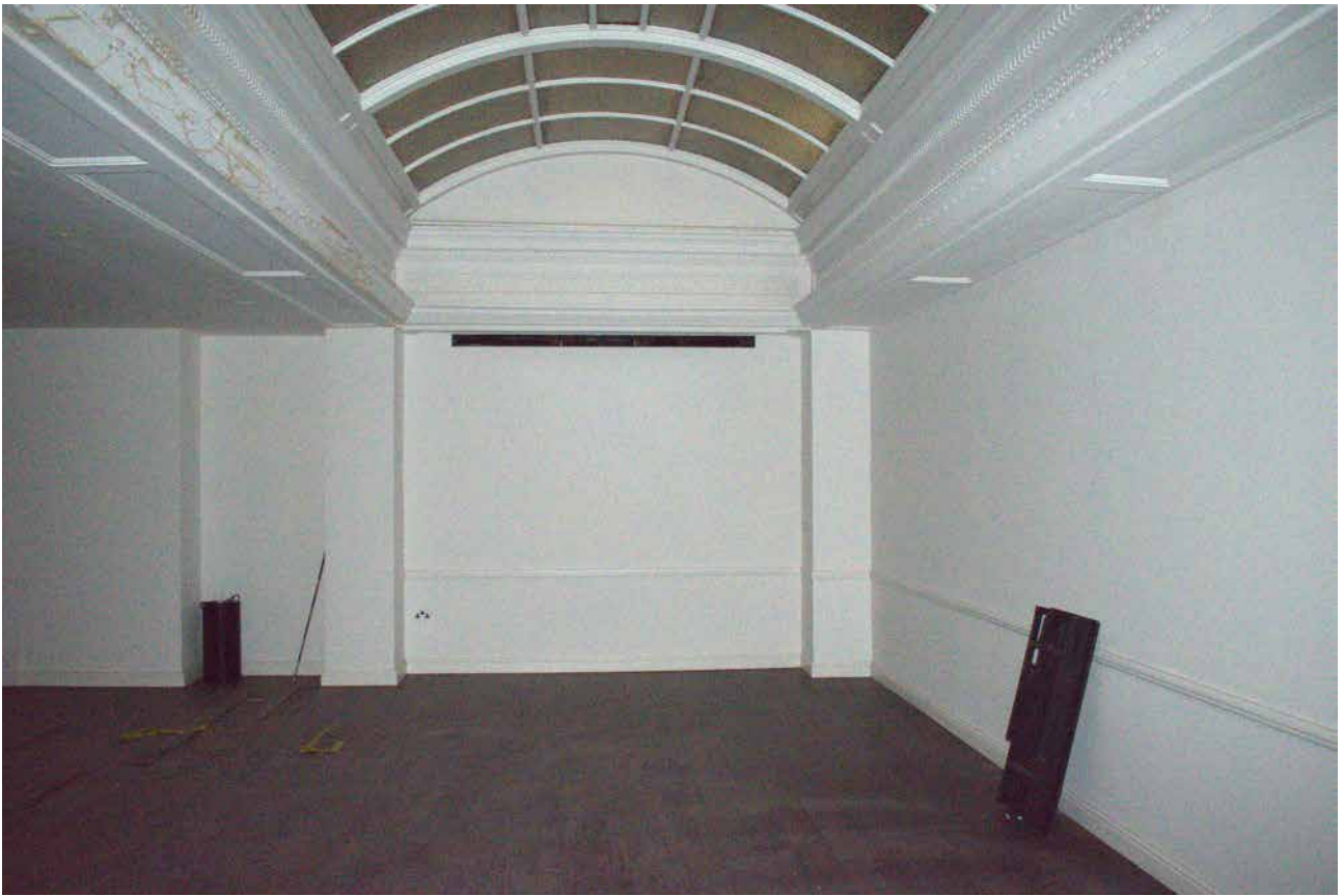
Plate 12 Rooflight illuminating the north part of the ground floor (DIA)
