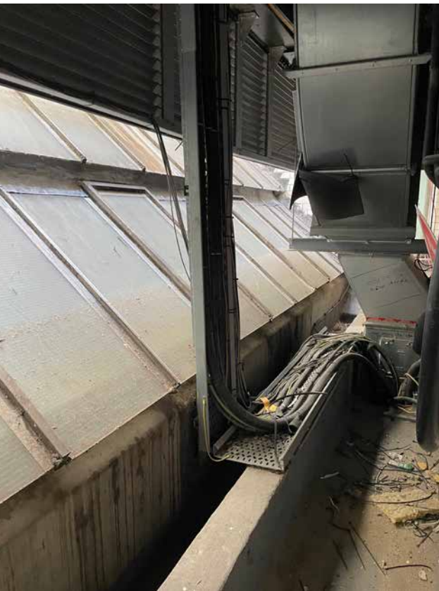
Plate 26 Glazed roof (north side) with gutter behind concrete parapet (DIA)
