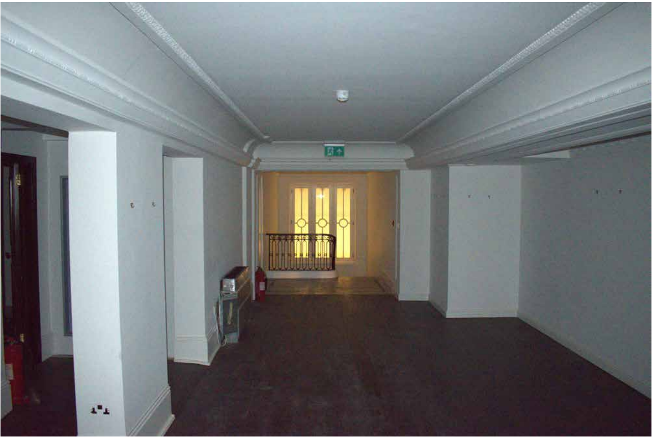
Plate 14 Mezzanine, looking west (DIA)
