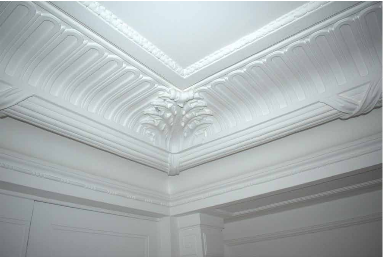
Plate 19 Cornice corner detail (DIA)
