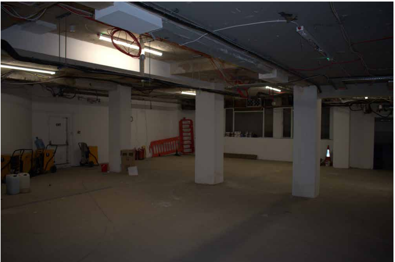
Plate 8 Basement, showing recent part-fit out works (DIA)
