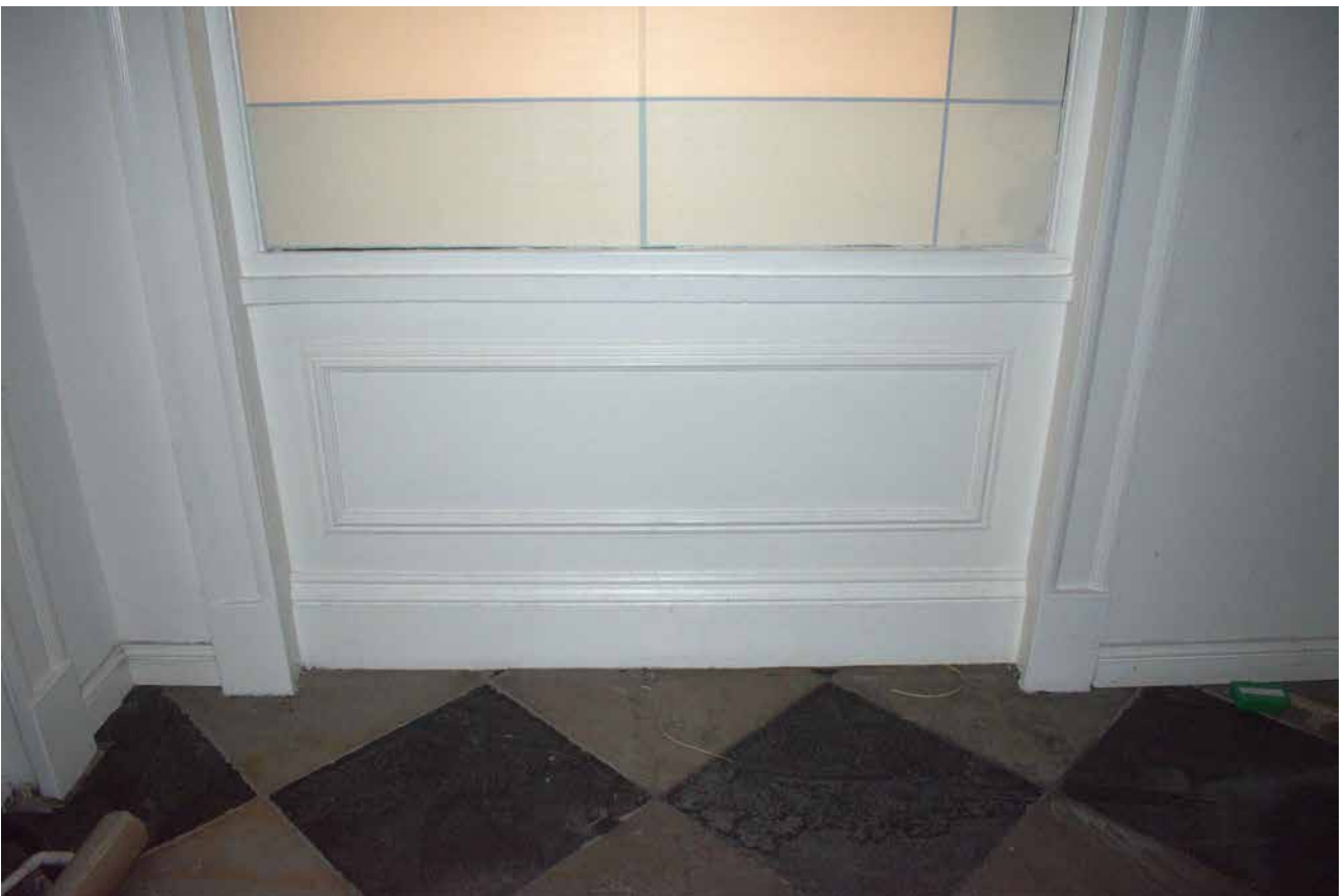
Plate 23 Panelling under ground-floor window (DIA)
