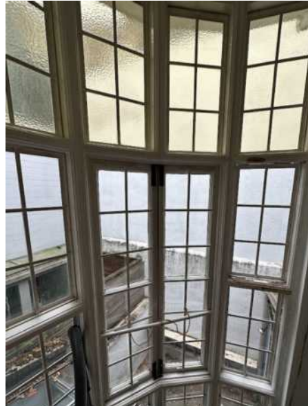
Fig 6: Curved Glazing at Rear
