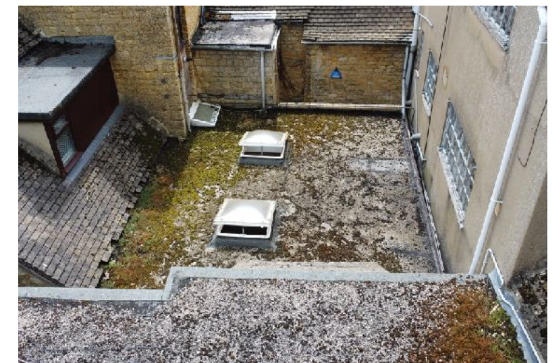
Existing modern flat roof courtyard extension
