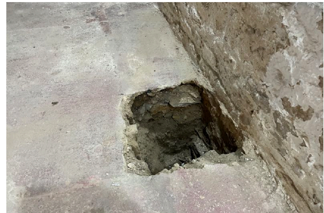
Damp concrete floor trial hole confirming underpinning walls is not required
