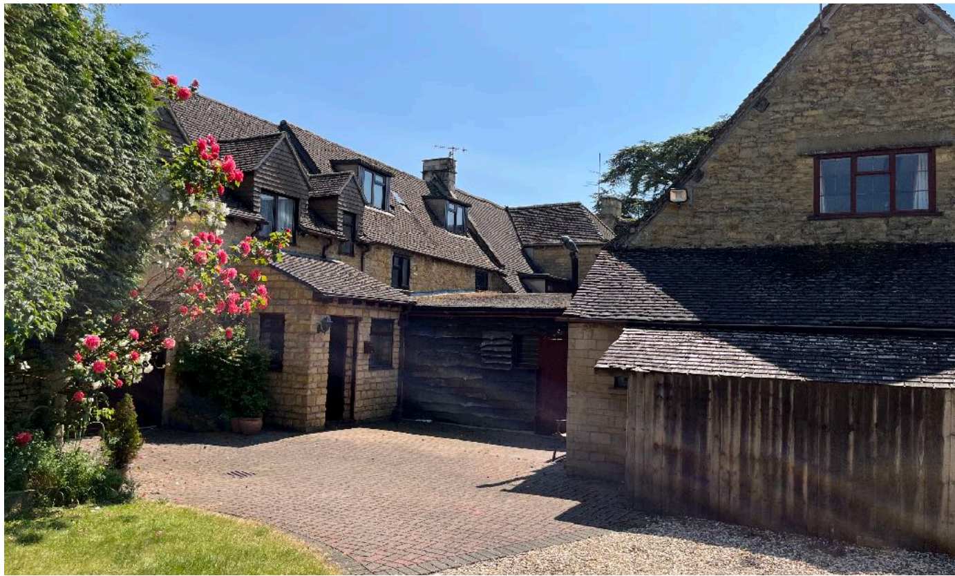
Photo of existing rear courtyard
