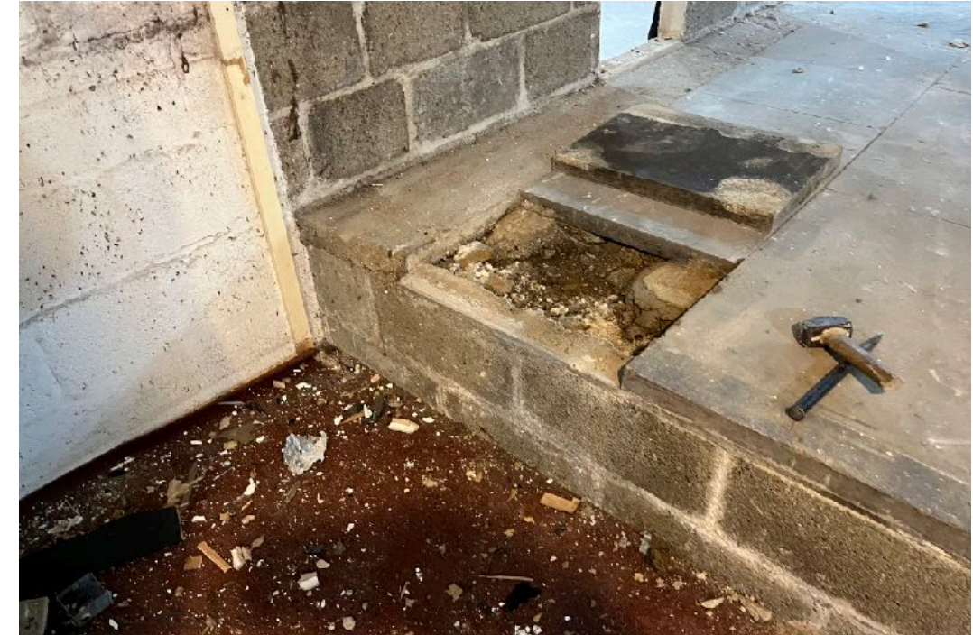
Modern floor in the courtyard extension
