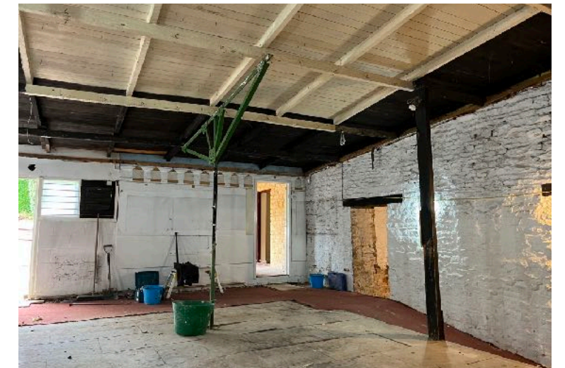
Existing courtyard extension to be demolished
