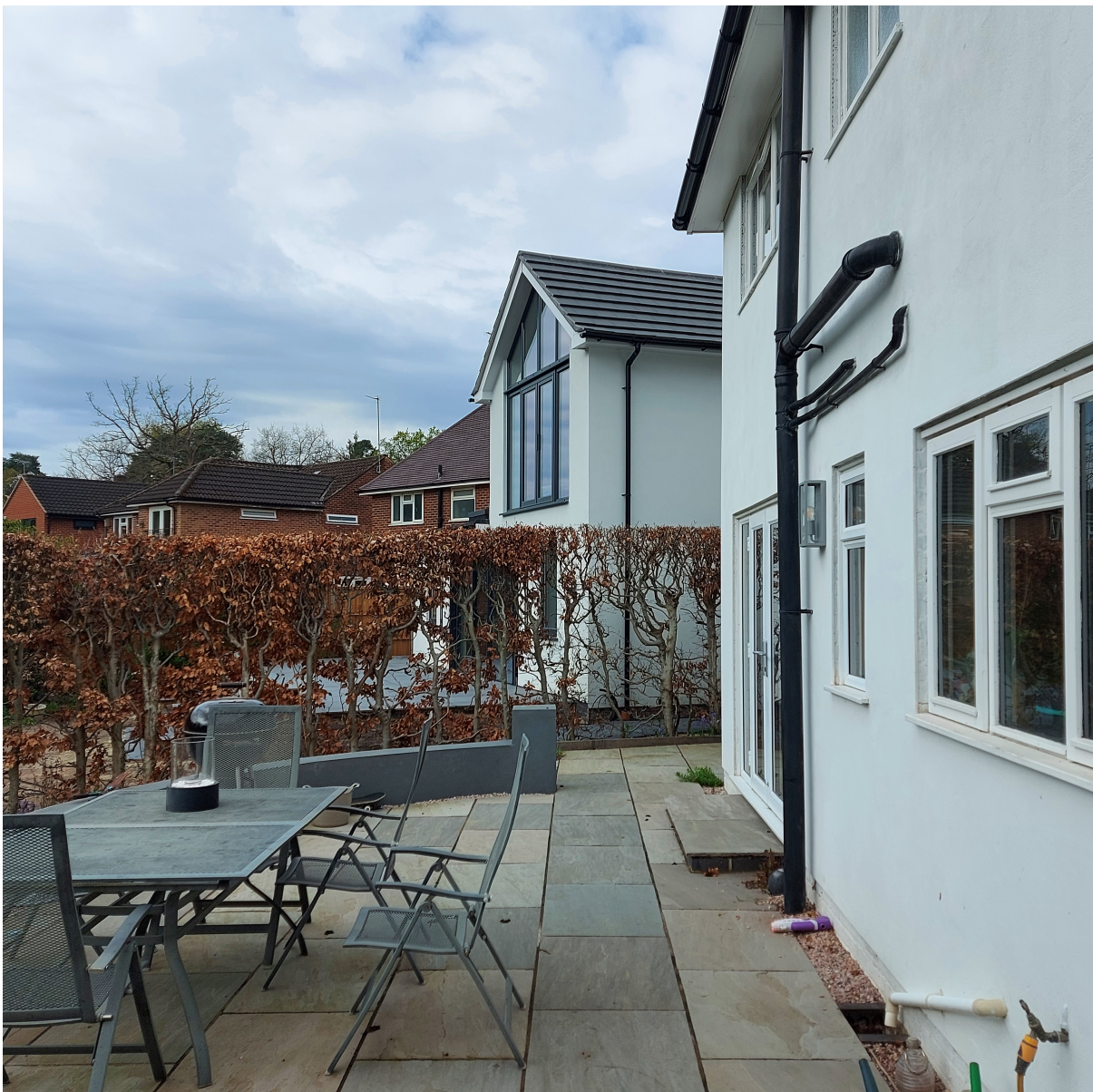
Photo 4: House 527 rear elevation showing gable roof design.
