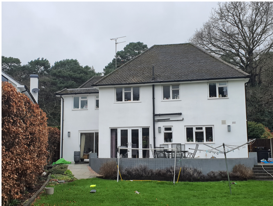
Photo 3: House #525 showing render finish to the rear.
