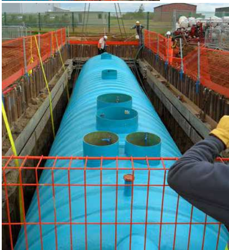
SPEL Separator being installed at an RAF base.
