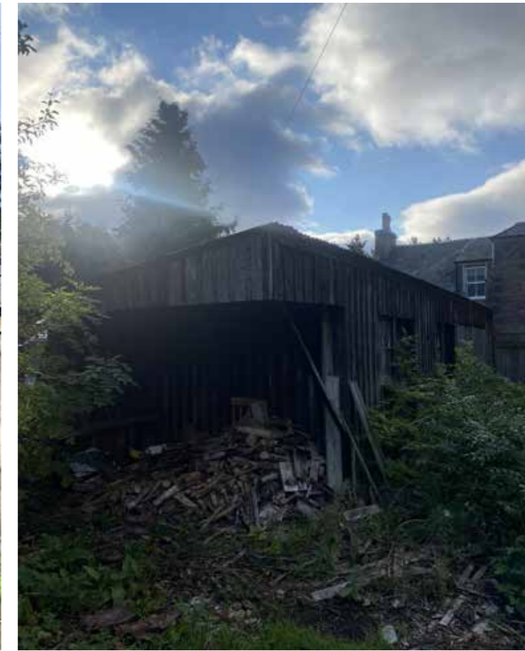
2. Photograph of existing timber sheds
