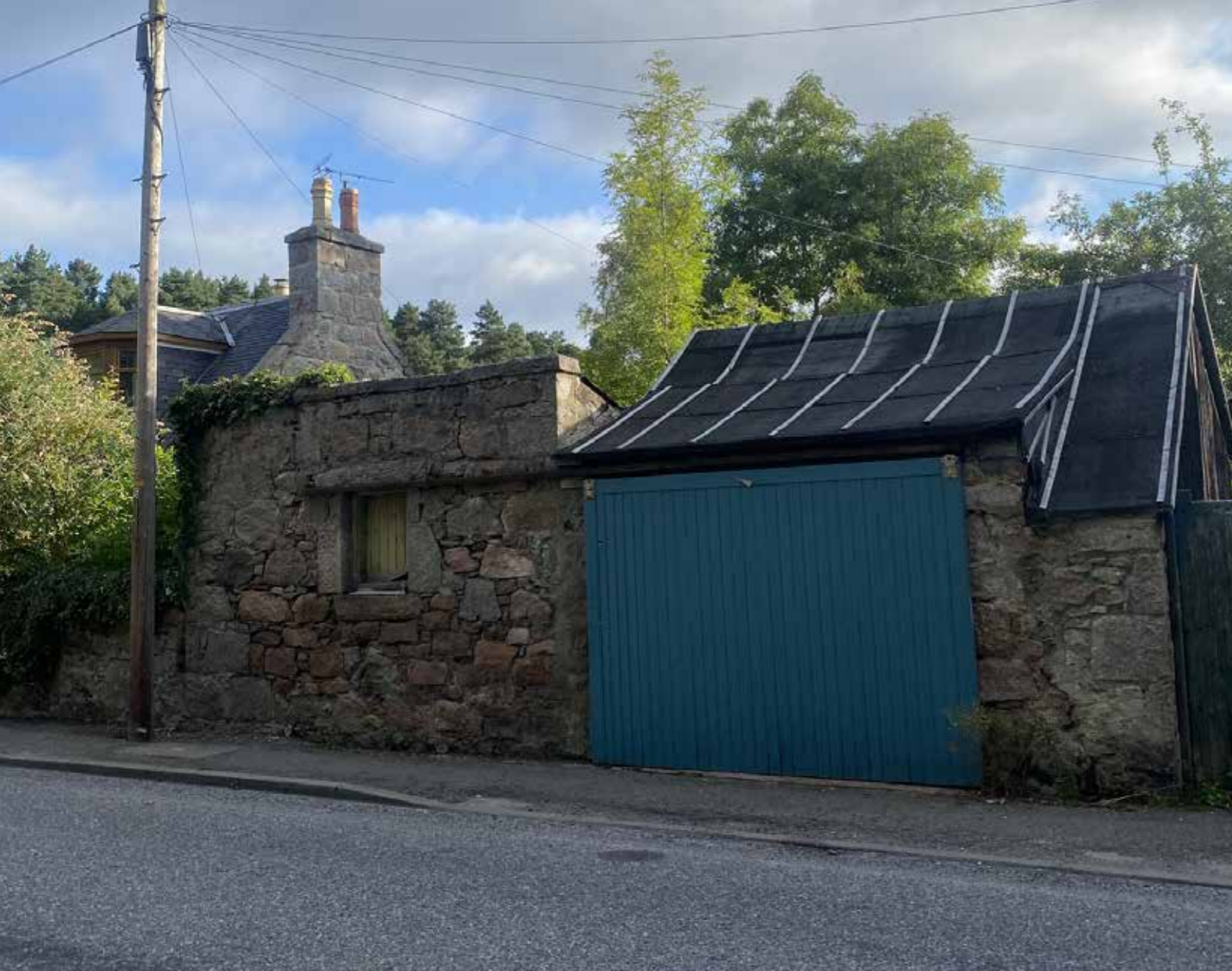
Photograph of existing garage and boundary wall
