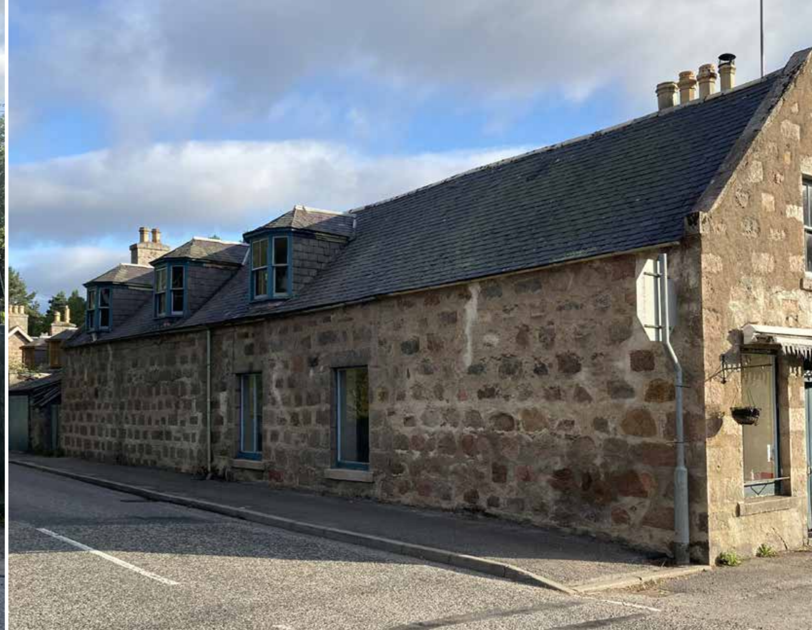
Photograph of West Elevation
