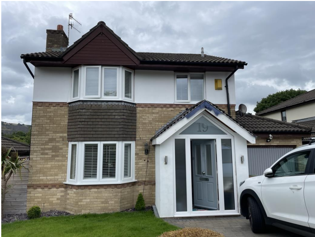
Fig 1 Front of property
