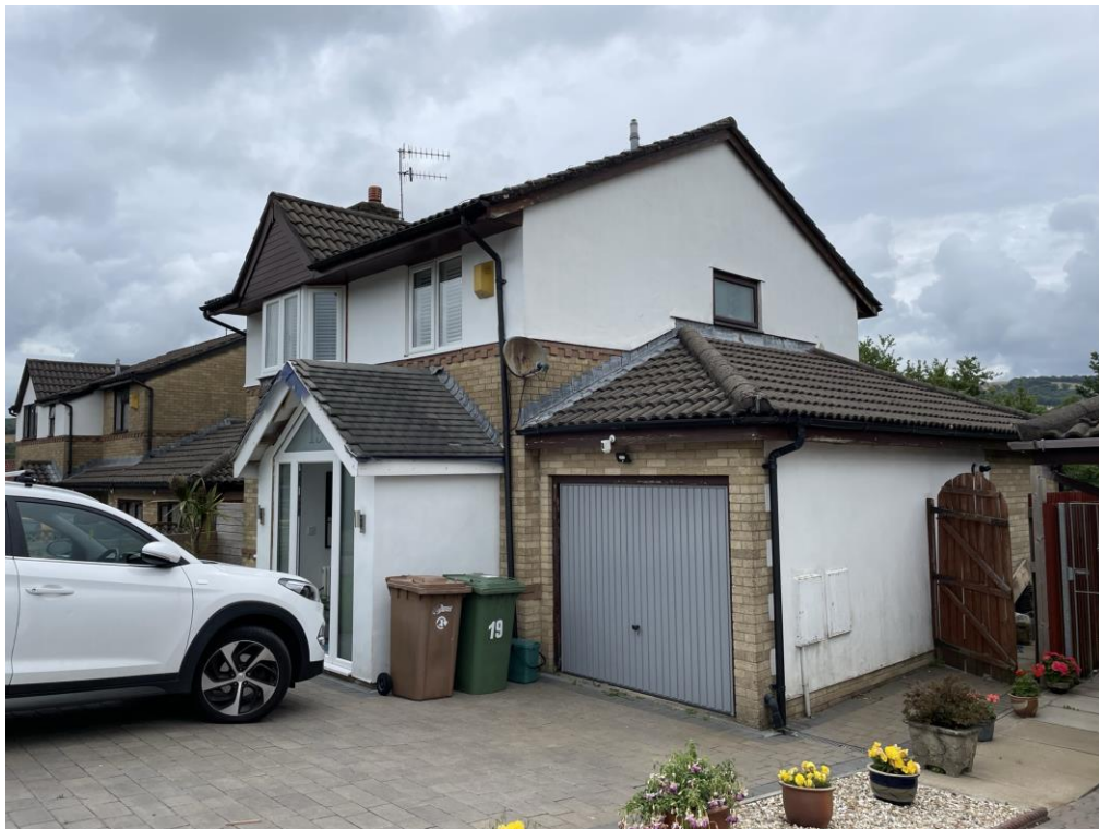
Fig 3 Side of property
