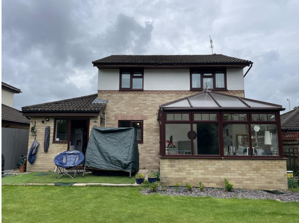
Fig 2 Rear of property
