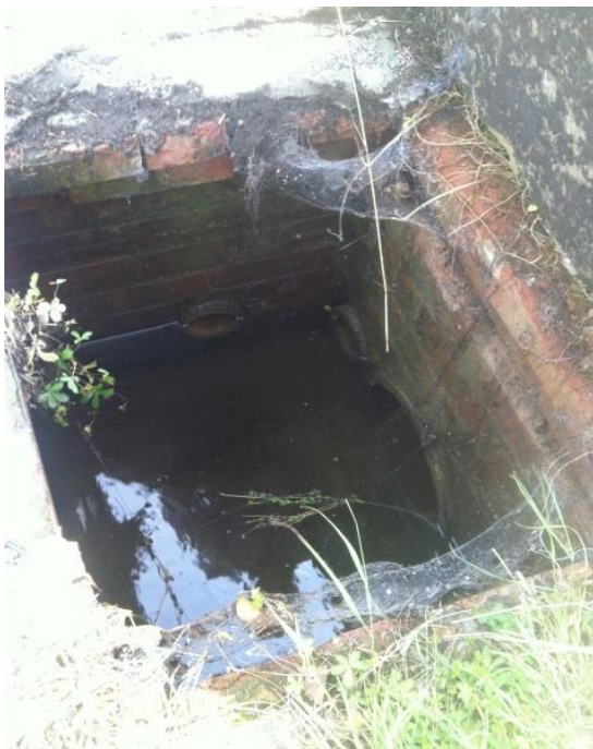
Figure 1.4: North End Stream Culvert at front of Bleak Farm property
