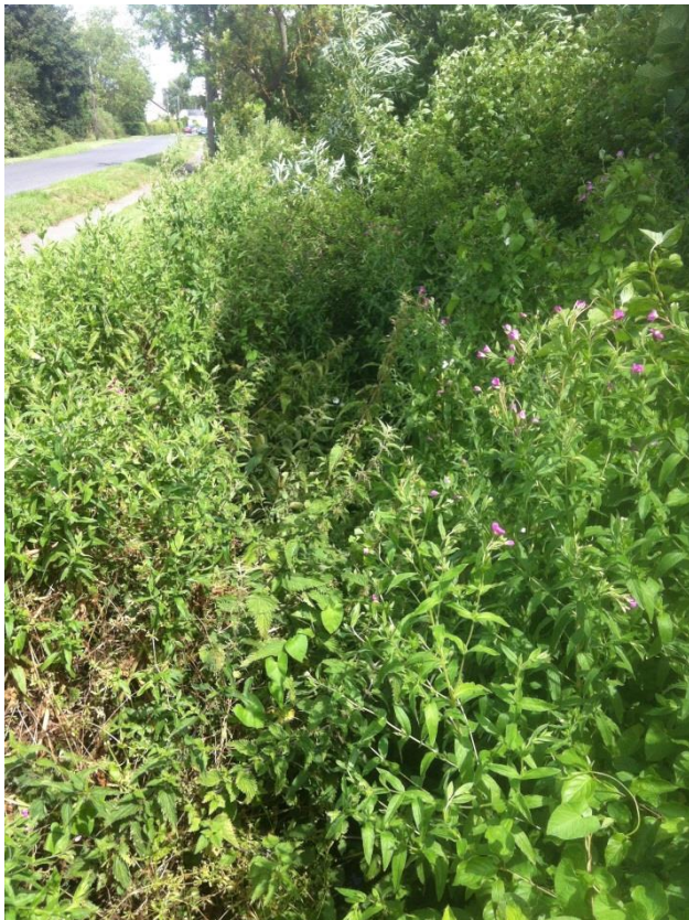
Figure A.7: North End Stream (facing d/s, prior to culvert under front of Bleak Farm)
