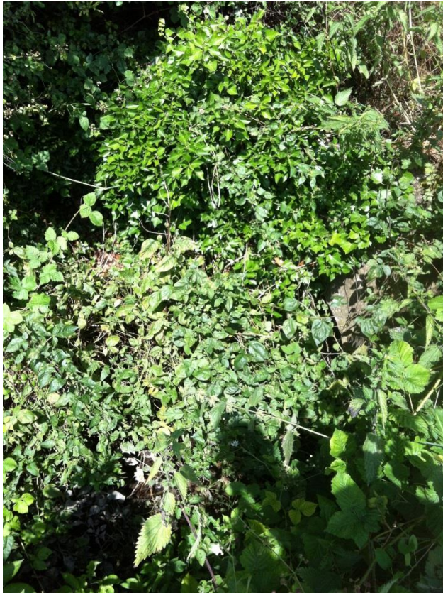
Figure A.3: Back Path Stream Culvert (d/s from Bleak Farm)
