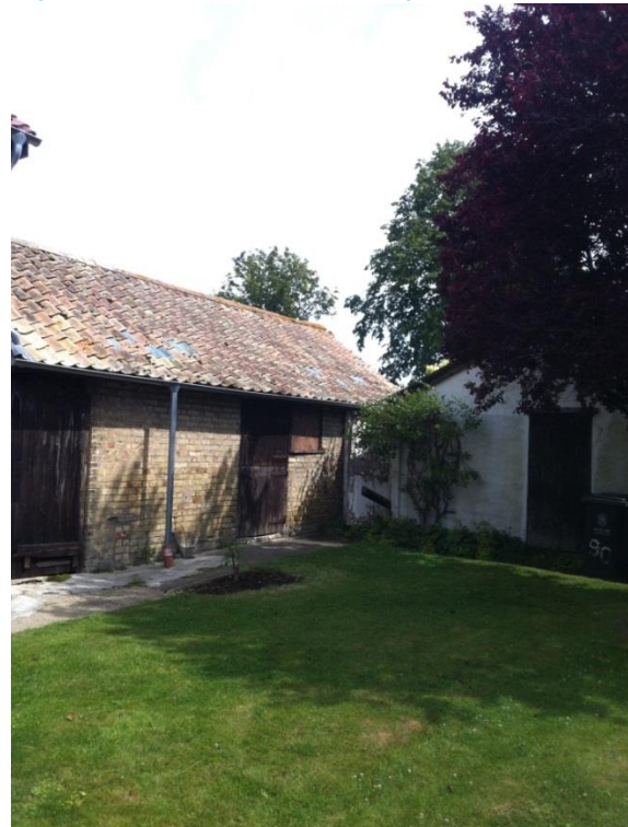
Figure 1.3: Site 2 – Small Storage Unit
