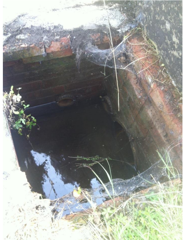
Figure A.6: Culvert under front of Bleak Farm
