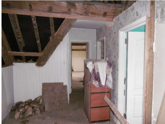
Modern partition on right hand side to be retained
