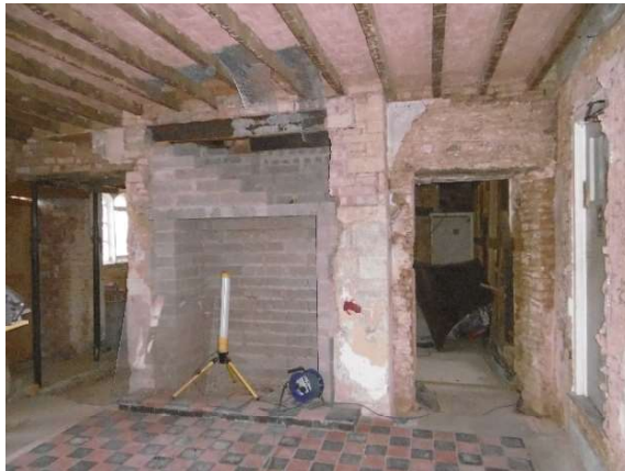
Reinstate fireplace in snug, work commenced.
