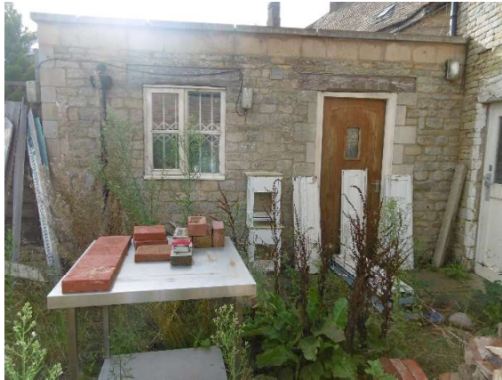
Modern flat roofed extension on the rear
