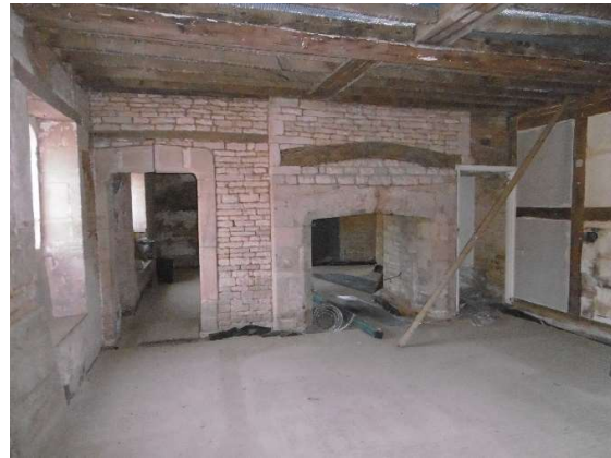
Retain un-plastered cross plasterboard new plasterboard ceiling
