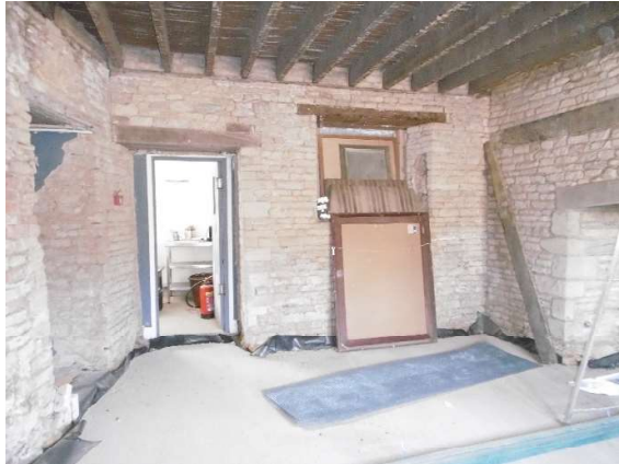
Block up modern door opening, new ceiling
