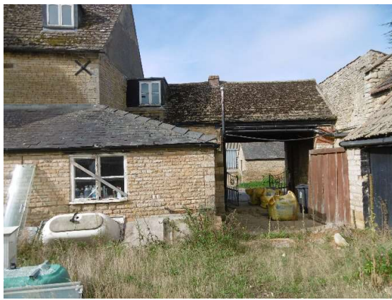
Modern lean-to extension on the rear
