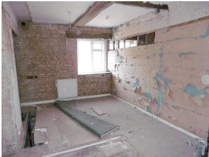
Bedroom 2 with central partition to be retained and ceiling to be made good
