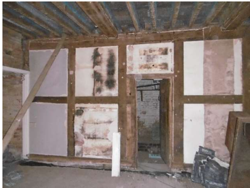
17 th century timber screen in dining room to be renovated
