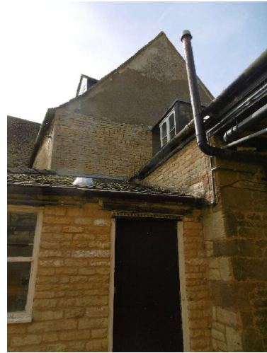
Northern gable to be rebuilt
