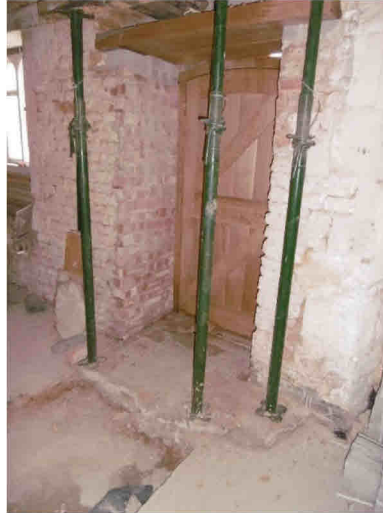
oak lintels to front door, X7
