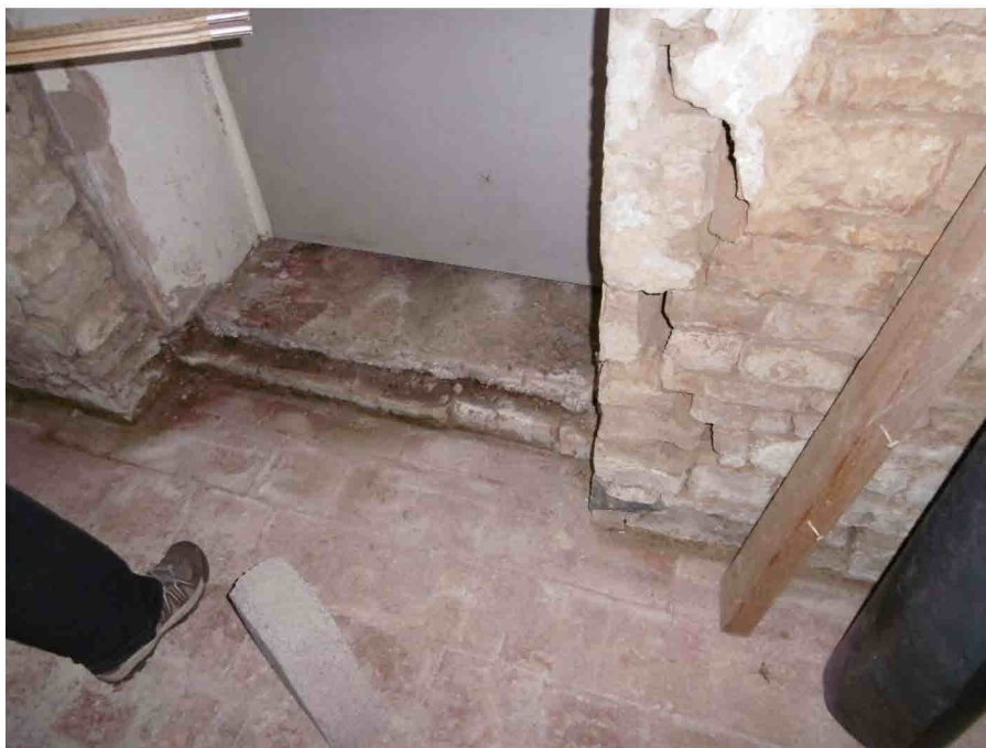
X3 Masonry pulling apart to RH side of door opening
