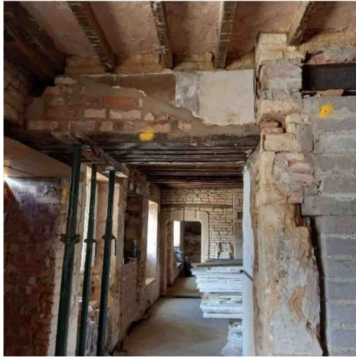
Timber lintels over opening, X6
