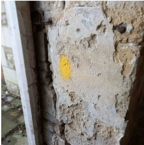
X3 Masonry pulling apart to RH side of door opening
