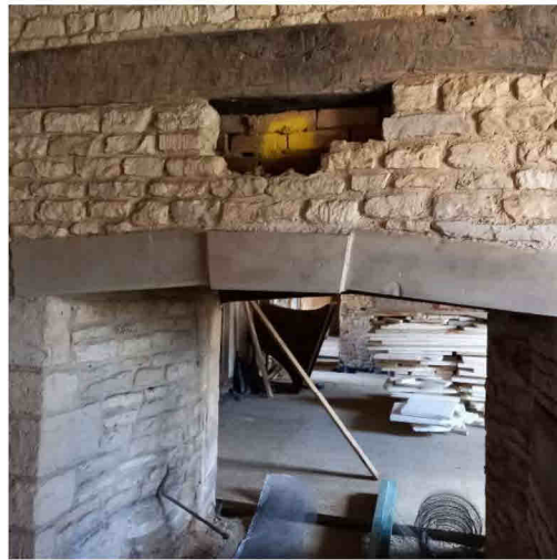
Lintels over fireplace
