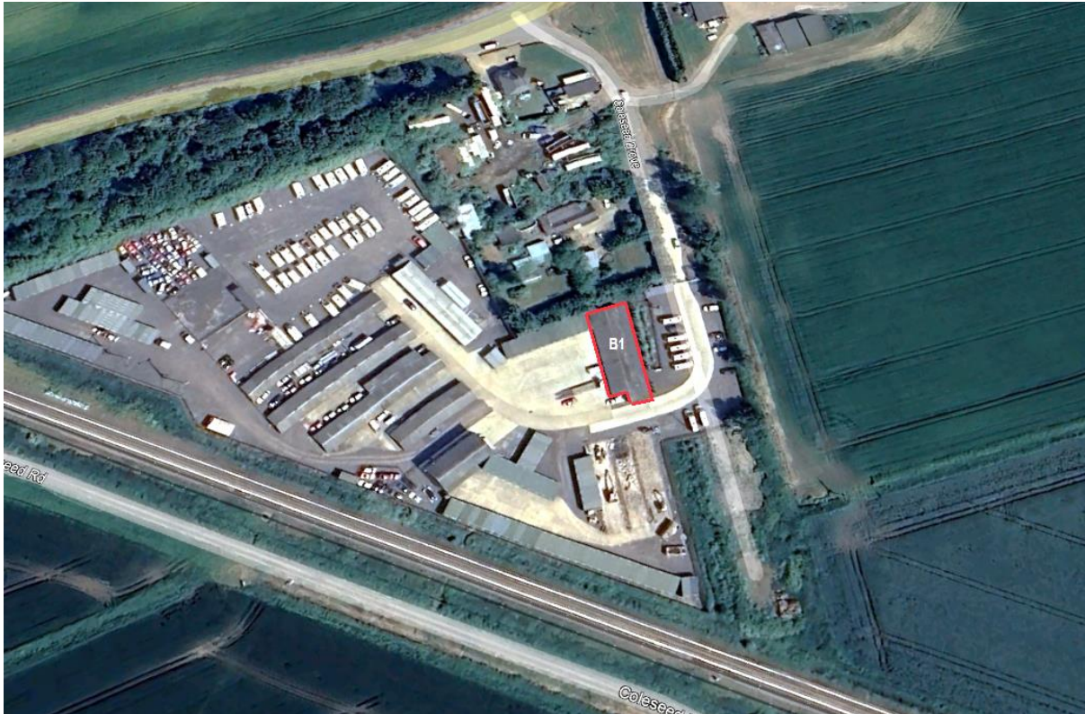
Fig 2. Aerial Site View and Buildings – Google Earth-June 2023
