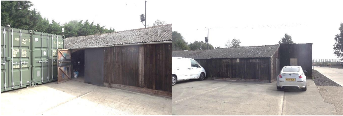
Fig 5. West elevation doors into units
