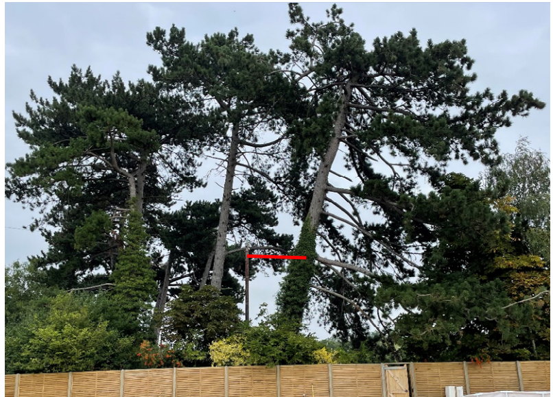
Photo 2: Pine tree T1 with current lean which has increased since 2017.
