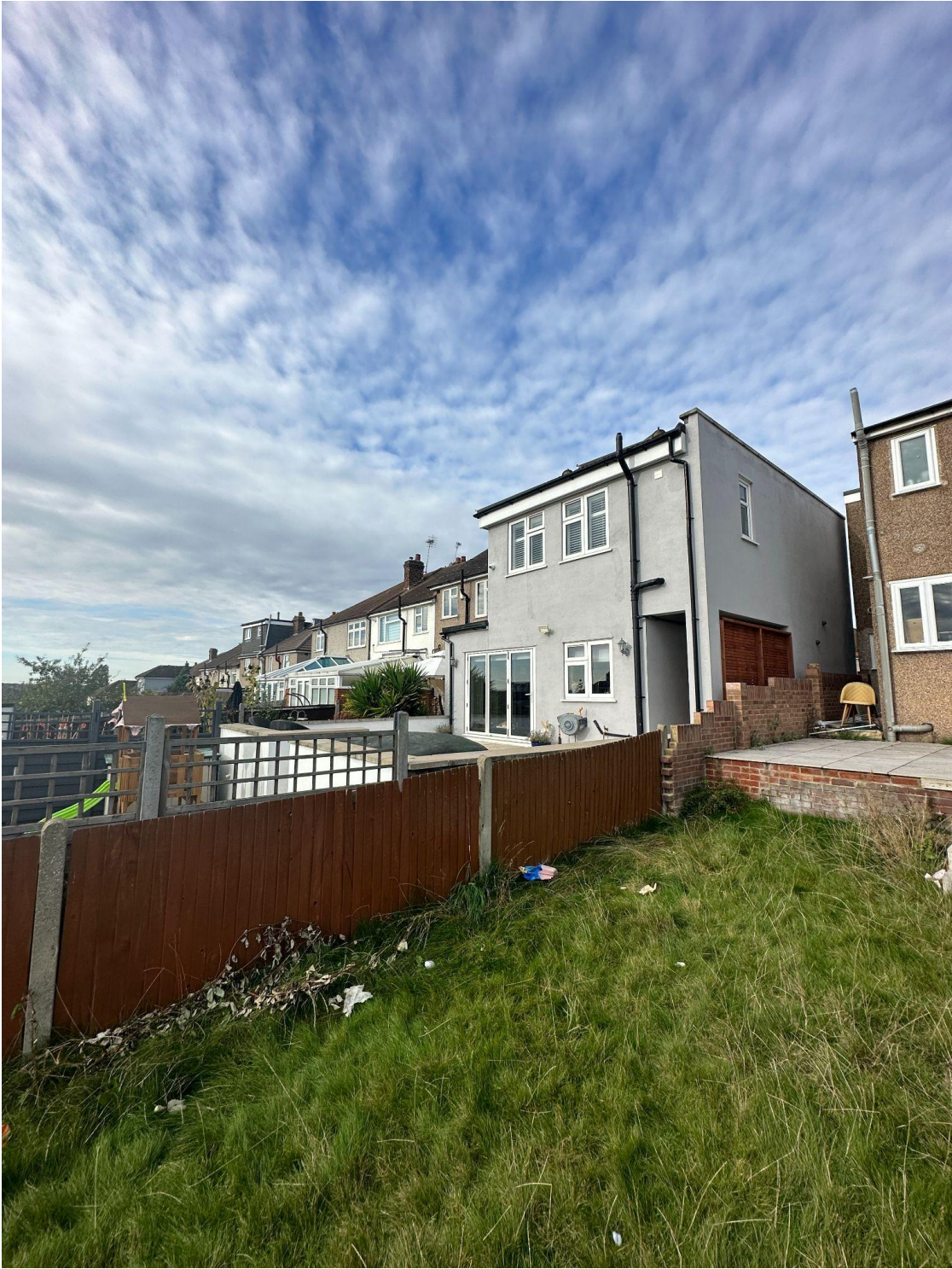
Image 03 - Rear View of 7 Somerset Avenue
