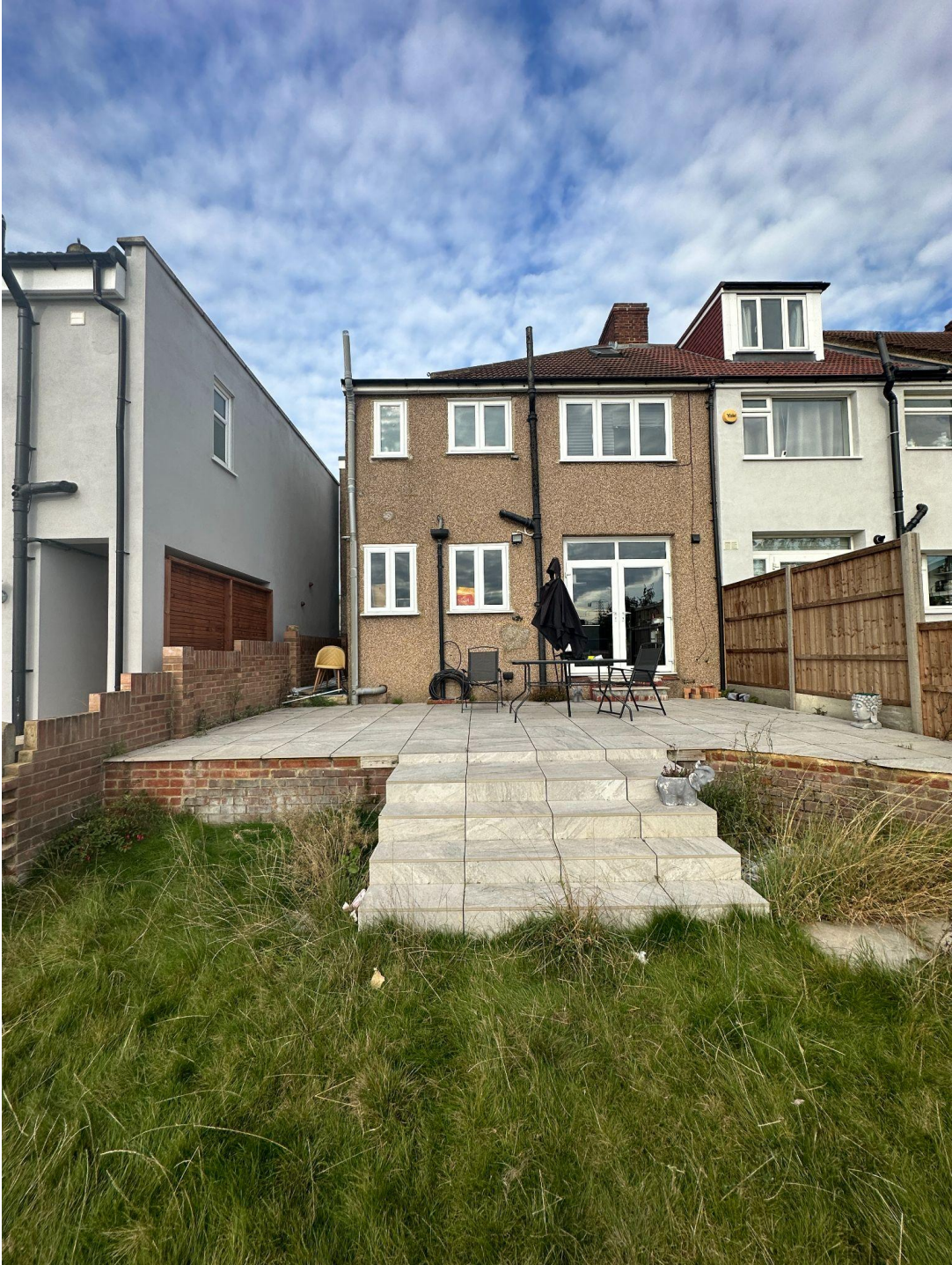
Image 02 - Rear View of 7 Somerset Avenue
