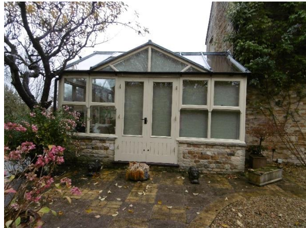
West elevation of conservatory
