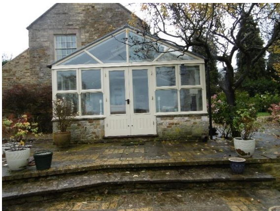
North elevation of conservatory
