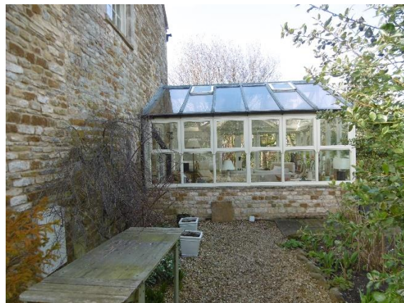
East elevation of conservatory
