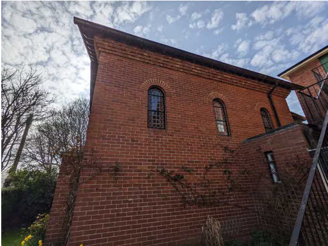
Photographs of chapel section within the Covent meeting, with decorative, stained glass windows to be replaced with matching timber double glazed units.
