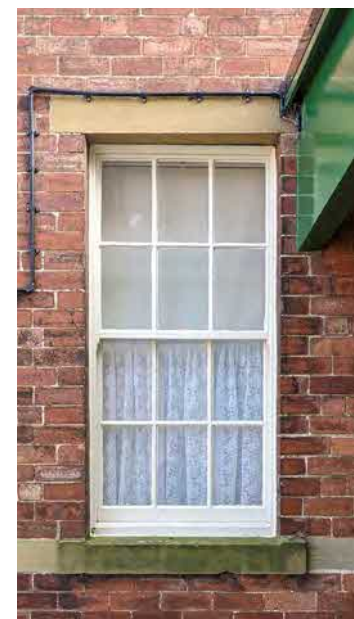
Examples of sash windows with brick pillar between, typical of the majority of windows on the main building, with a six-over-six window pane arrangement
