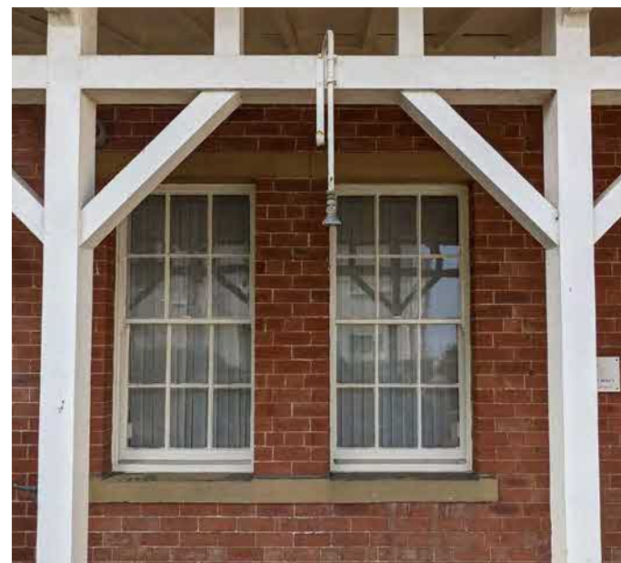
Examples of sash windows with brick pillar between, typical of the majority of windows on the main building, with a six-over-six window pane arrangement
